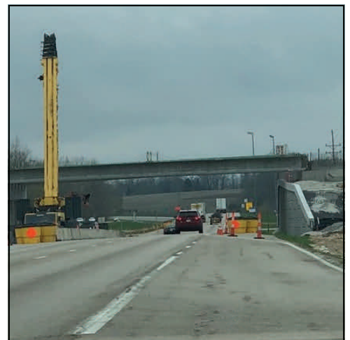
Girders for the Route P/Peine bridge
