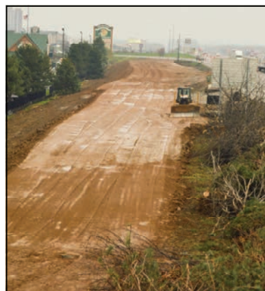
Construction of new ramp at I-70 and Fairgrounds Road.
