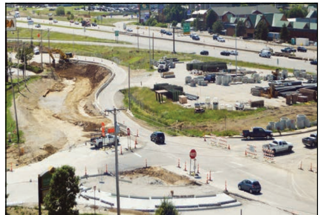
Roundabout construction at Veterans Memorial Parkway and Fairgrounds Road.
