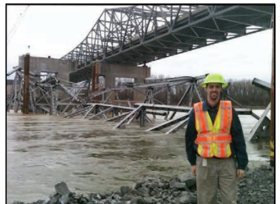
At the Demolition of the Blanchette Bridge
