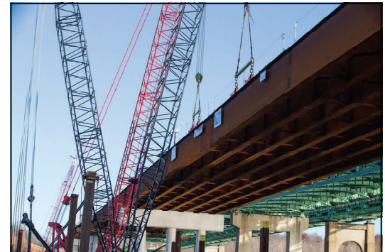
Crews set the final girder for the new Boone Bridge.
