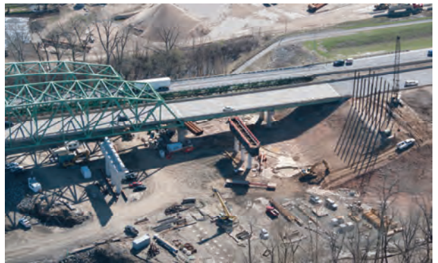
Aerial view of foundation work on the new bridge.
