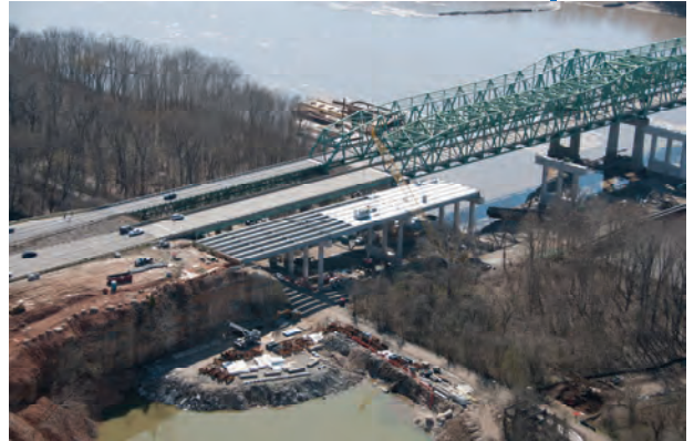
Aerial view of new bridge from the St. Charles side of the river.
