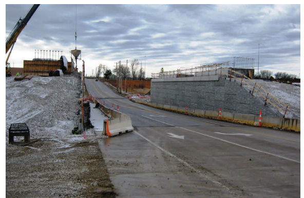
New bridge walls going up at Henke Road as part of the Route 364 Page Phase 3 project.
