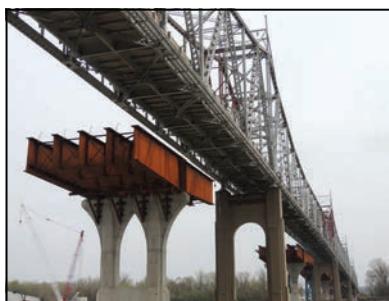
Bridge girders set behind current bridge.
