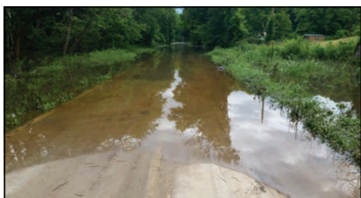
Flooding on Route AA in Jefferson County
