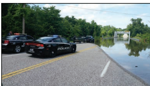
Flooding on Route 61 north of Herculaneum
