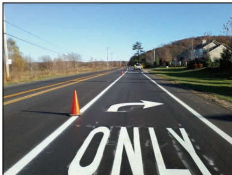
Turn lanes were added on portions of Route W in 2014, including at Mirasol Manor.
