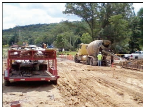
Crews working on safety improvements on Route W last year near the Fox Run Golf Club.
