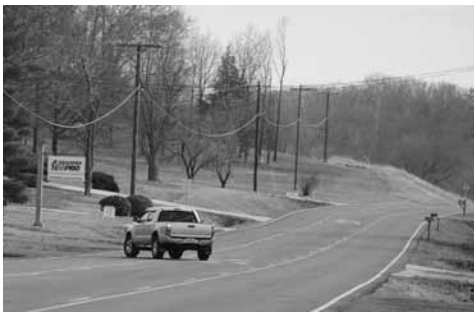
With the major work completed, drivers are utilizing the newly improved Route 34. Additional work will be completed on the St. Francis River Bridge and a bridge on County Road 219 near Silva.
