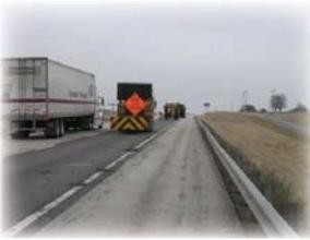
These operations often involve frequent, short stops for activities where workers are on foot. **These stops can only last up to 15 minutes in duration.** Typical work activities include litter cleanup and pothole patching.
