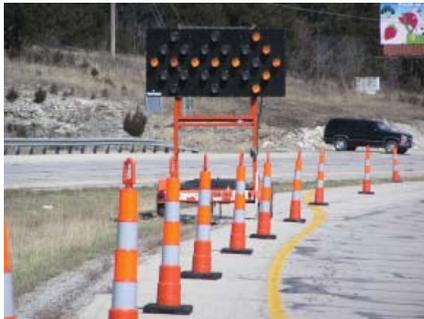
For stationary lane closures, the panel should be deployed on the shoulder or within an adjacent closed lane at the beginning of the lane or one-lane, two-way taper. Where adequate space or the temporary traffic control plan does not permit this placement, the unit may be placed within the taper of the closed lane. When closing multiple lanes, a separate unit shall be used to close each lane.
