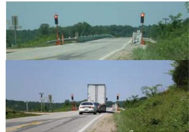
**RC Flagman-**The mechanical flagger system consist of a red and amber indication signal head, and a PVC flagger arm. The RC Flagman is placed at one end of the work zone substituting one human flagger, and is remotely controlled by a human flagger located at the other end of the work zone.
