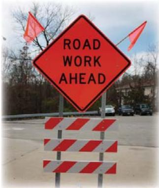
used to enhance the target value of certain signs on long-term stationary operations. The AWRS is only installed on the first occurrence of the ROAD/BRIDGE WORK AHEAD (WO20-1) signs on the mainline roadway.
