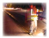
lighting, as described in Section 616 of the EPG. Work zone lighting is specified on the plans and is included as a pay item when work is required at night or when lighting needs to be present during non-working hours (i.e. lighting gore areas, crossovers, etc.).
