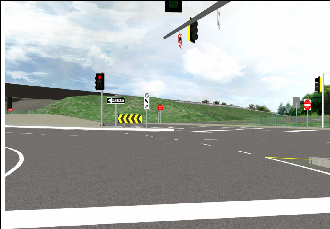
Figure 6. The crossover on the eastern node of the interchange where drivers on the northbound offramp could see a path to the opposing eastbound lanes.
