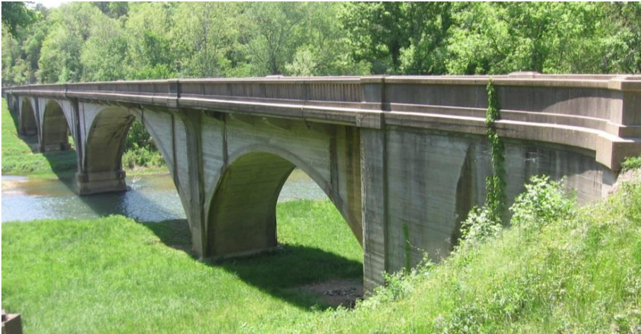
2. Current River Bridge
