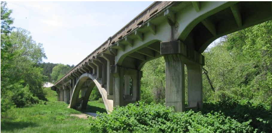
3. Round Spring Bridge over Spring Valley Creek
