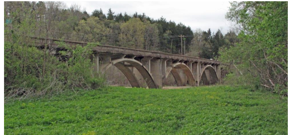
1. Sinking Creek Bridge
