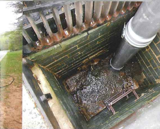
Powaboom option cleaning catch basin.
