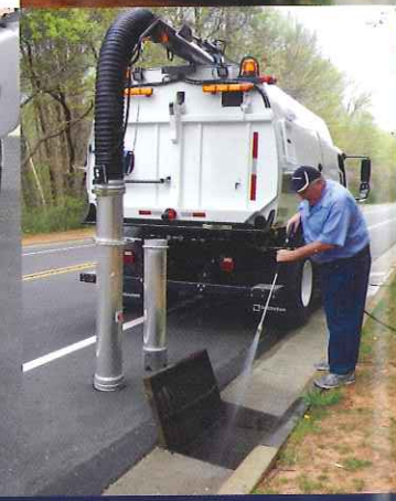
Supawash hand lance in action while servicing catch basin.
