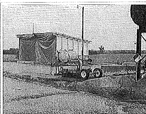
Salt and salt mix stored inside away from moisture. Note that surface water is diverted from the storage building.
