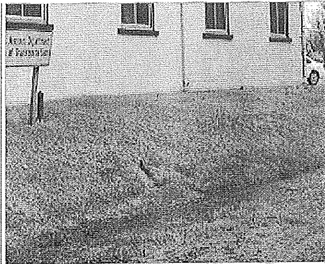
Floor drain discharges to road ditch
