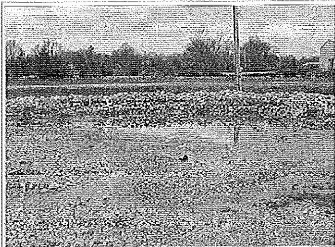
This berm hold the water long enough for the silt and suspended particles to settle and can be easily cleaned. It dries out between rains.
