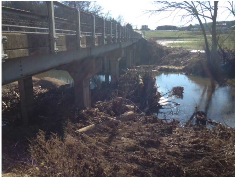
Location #4: Gasconade County, Rt A Bridge #X0984, at Crider Creek
