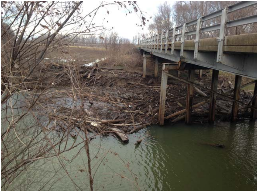
Gasconade County, Hwy 100 Bridge #L0321, at Bailey's Creek
