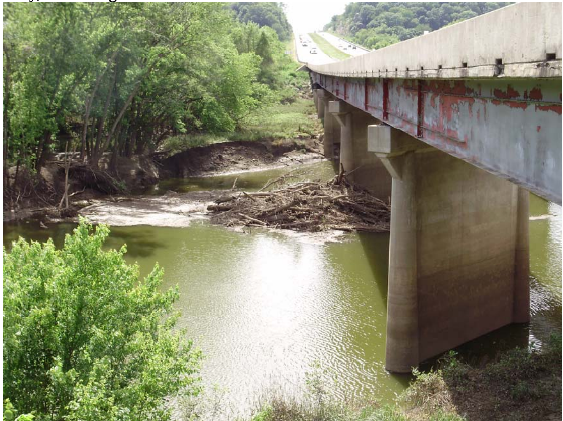
Cooper County, I-70 Bridge
