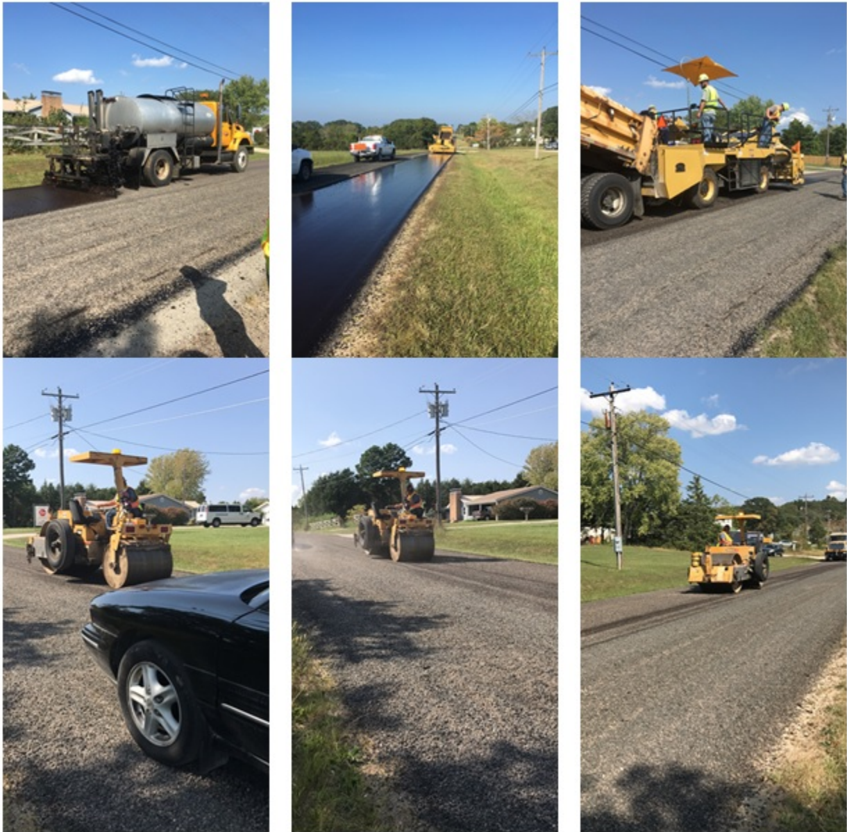
Figure C-17: Construction of field test sections
