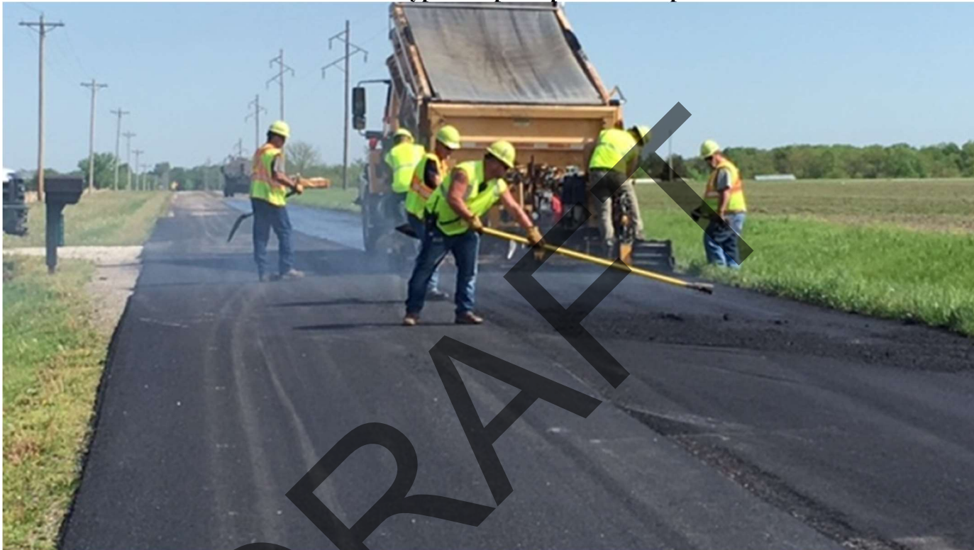
Typical asphalt pavement repair
