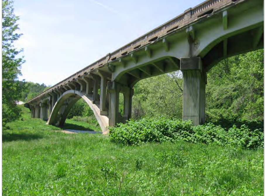
Shannon County Route 19 MoDOT Job No. J9P0438
