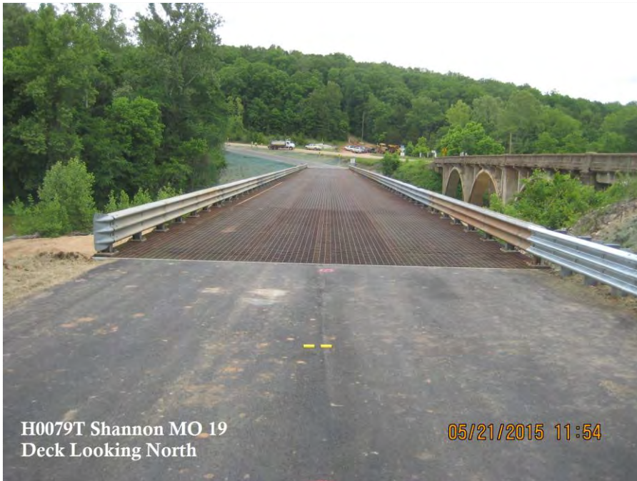
Sinking Creek Temporary Bridge (H0079T), facing north
