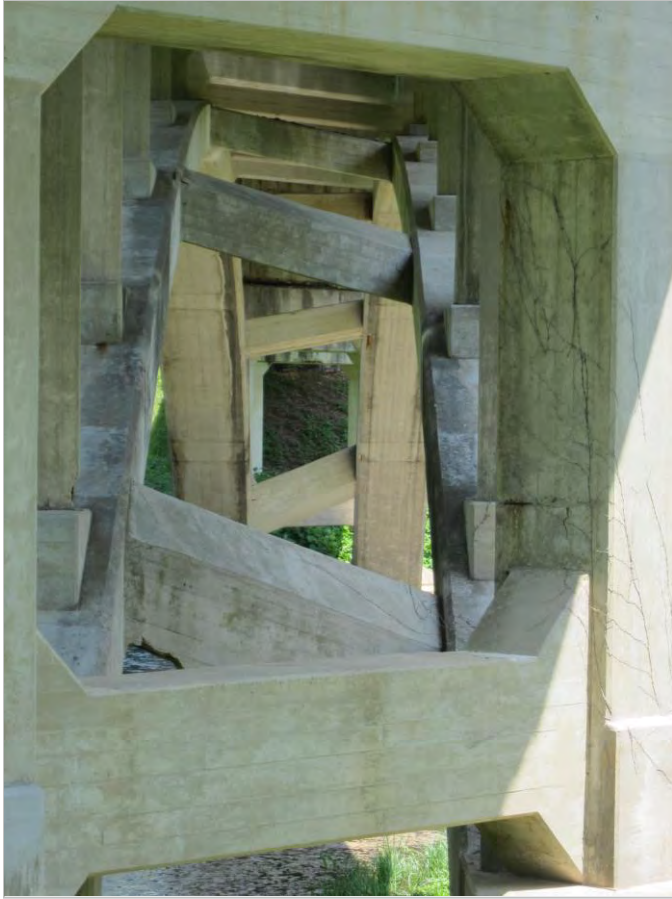
Spring Valley (Round Spring) Bridge (J0420), facing north
