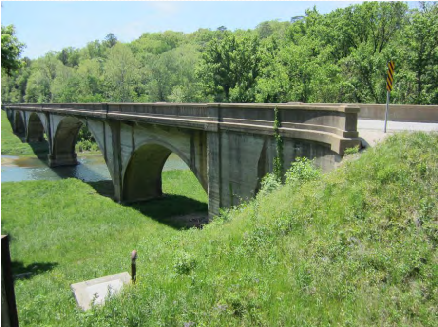
Current River Bridge (G0804), facing southwest
