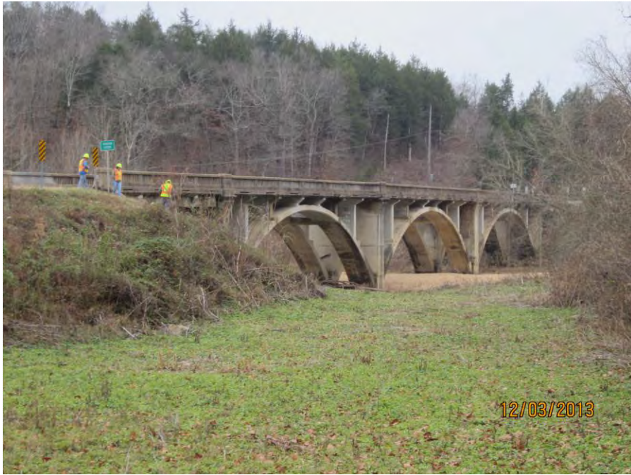
Sinking Creek Bridge (H0079), facing southeast
