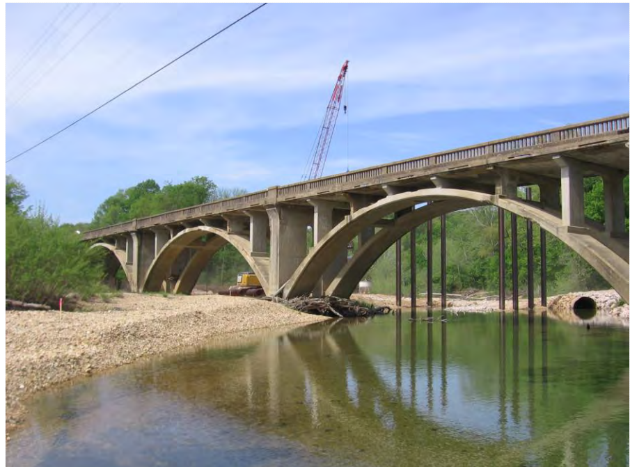
Sinking Creek Bridge (H0079), facing southwest
