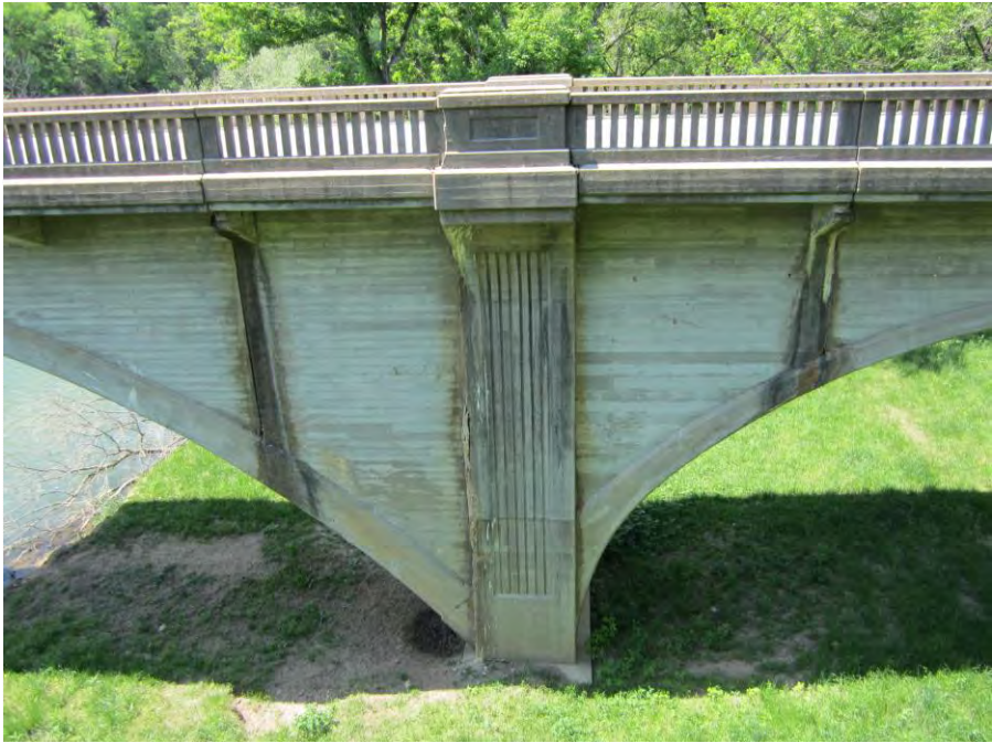
Current River Bridge (G0804), facing east
