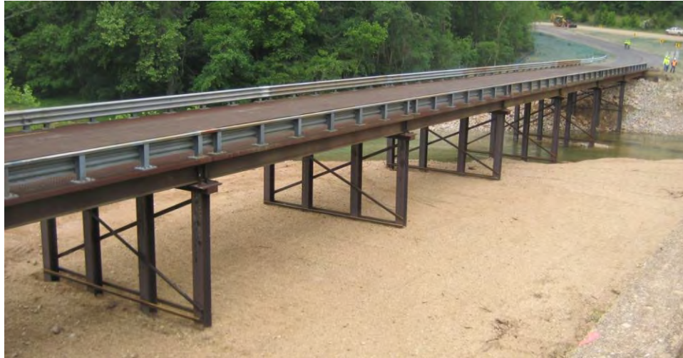
Figure 2: Temporary Bridge at Sinking Creek (2015)
