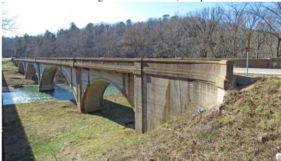
Figure 3: Current River Bridge (2015)
