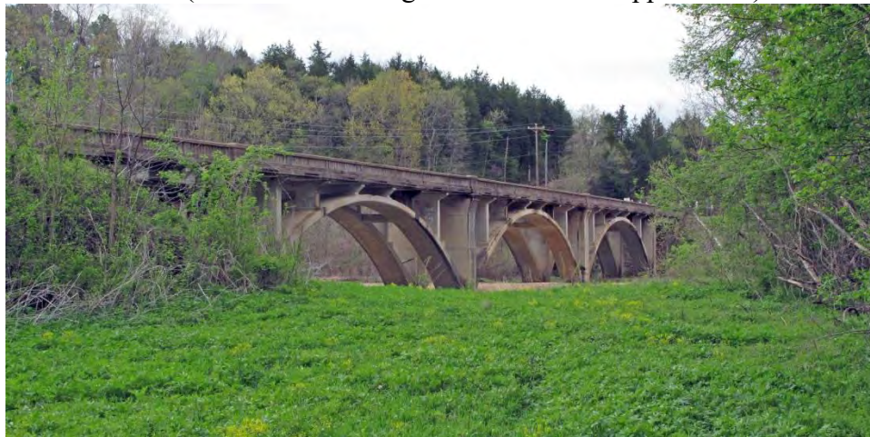
Figure 1: Sinking Creek Bridge (2015)
