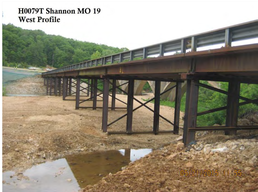
Sinking Creek Temporary Bridge (H0079T), facing north
