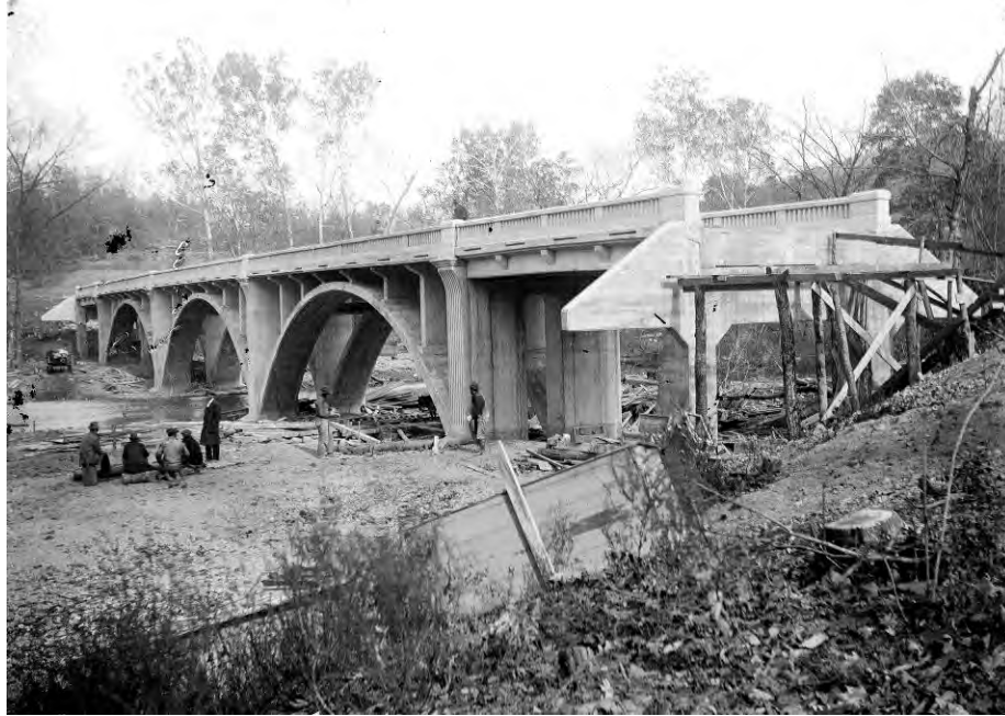
Figure 12: Sinking Creek Bridge during construction, (Gill 1926)
