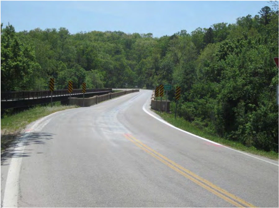
Current River Bridge (G0804), facing south
