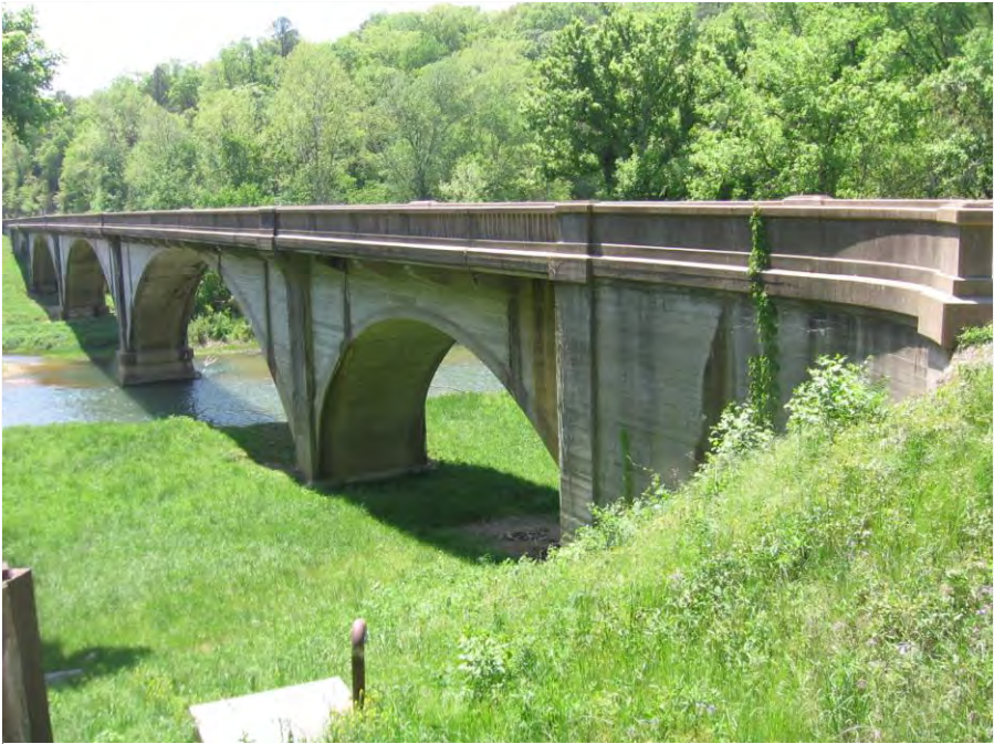
Current River Bridge (G0804), facing northwest
