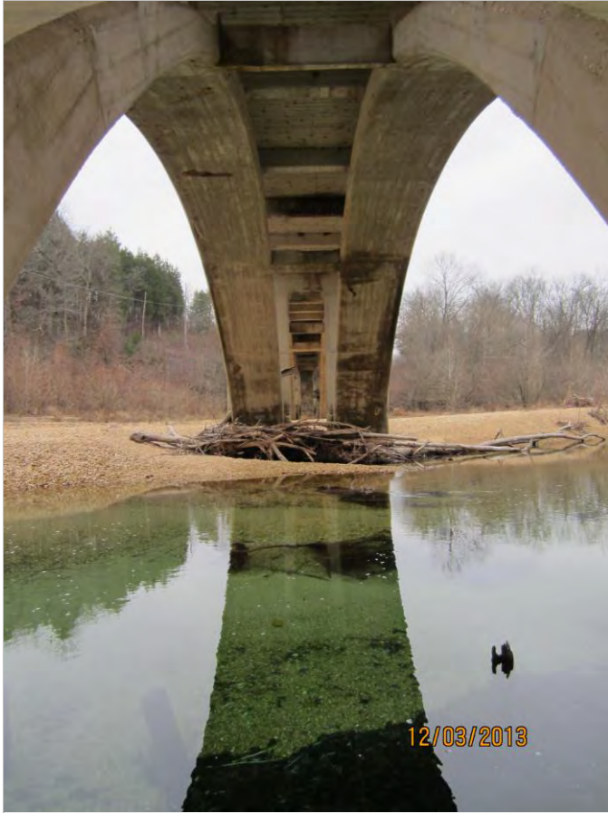
Sinking Creek Bridge (H0079), facing south
