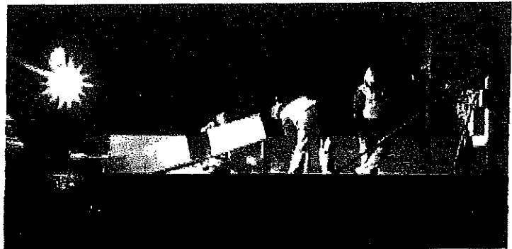
Crew takes a soil sample on an interstate to determine soil conditions and how much rock is beneath the surface.
