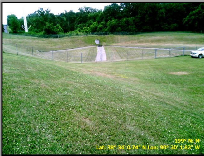
Figure 9: Permanent detention basin on Route 141 and Big Bend Rd.
