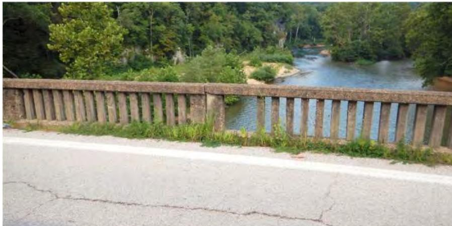
**Figure 8-2. Existing Current River Bridge Rail – Back Face with Post**
