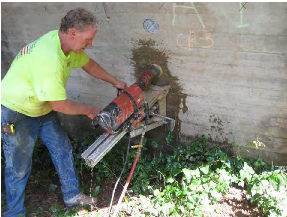
Photo 8: Concrete Coring
