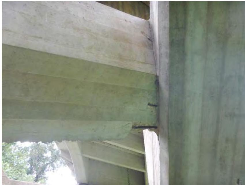
Lateral Bracing Between the Arch Ribs
