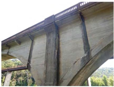
Leakage from Sidewall Joints
