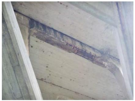
Typical Deterioration on Spandrel Capbeams
