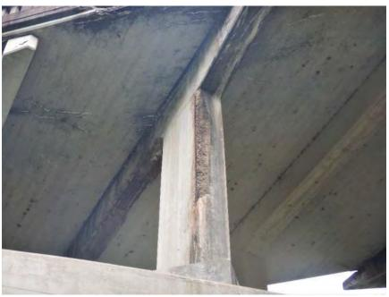
Typical Deterioration on Spandrel Columns
