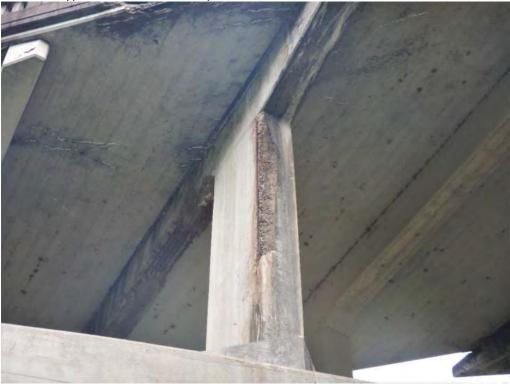
Pic. 009: Typical deterioration of spandrel column
