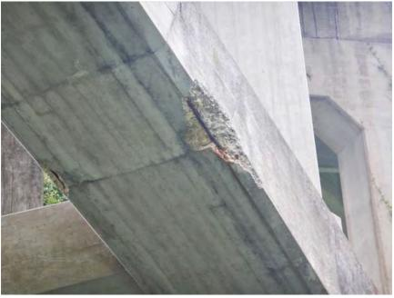
Spalling and Delamination of Arch Ribs
