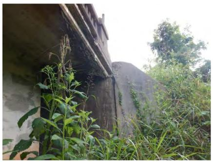
Typical Spalling at Abutment
