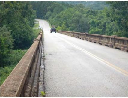
Collision Damage to the Railing
