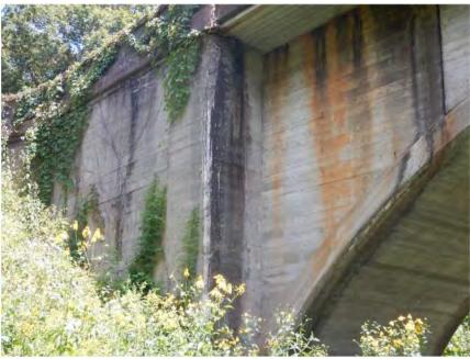
Cracking and Delamination at Abutments
