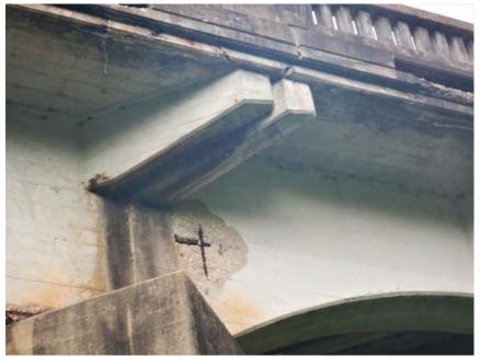
Typical Delamination on Girders
