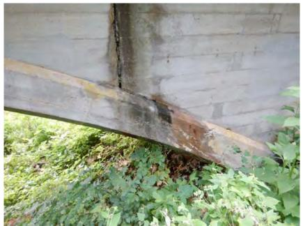
Spalling and Staining on Arch Ring
