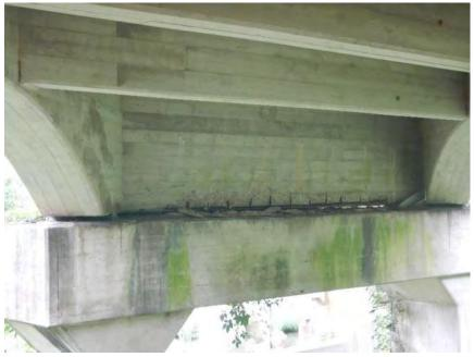
Deterioration of Floorbeams at Intermediate Bents
