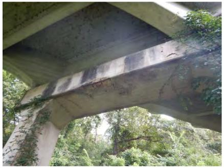
Deterioration of Intermediate Bent Cap Beams
