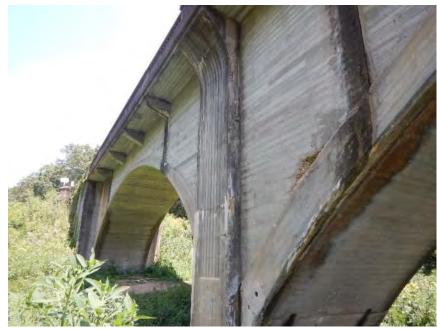
Spalling on Pier Surfaces
