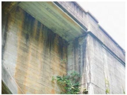
Typical Spalling at Abutment Corners
