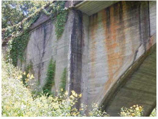
Pic. 007: Cracking and delamination, Abutment 1 west side
