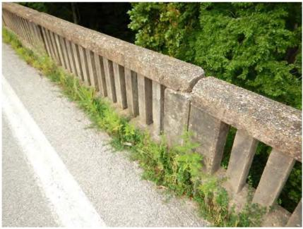
Collision Damage to the Railing
