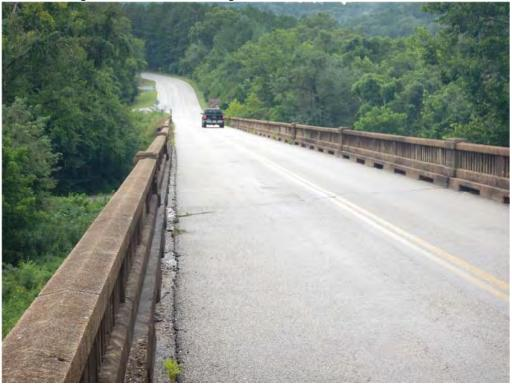
Pic. 003: Bridge barrier rail with misalignment
