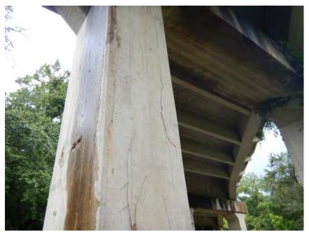
Deterioration of Intermediate Bent Columns
