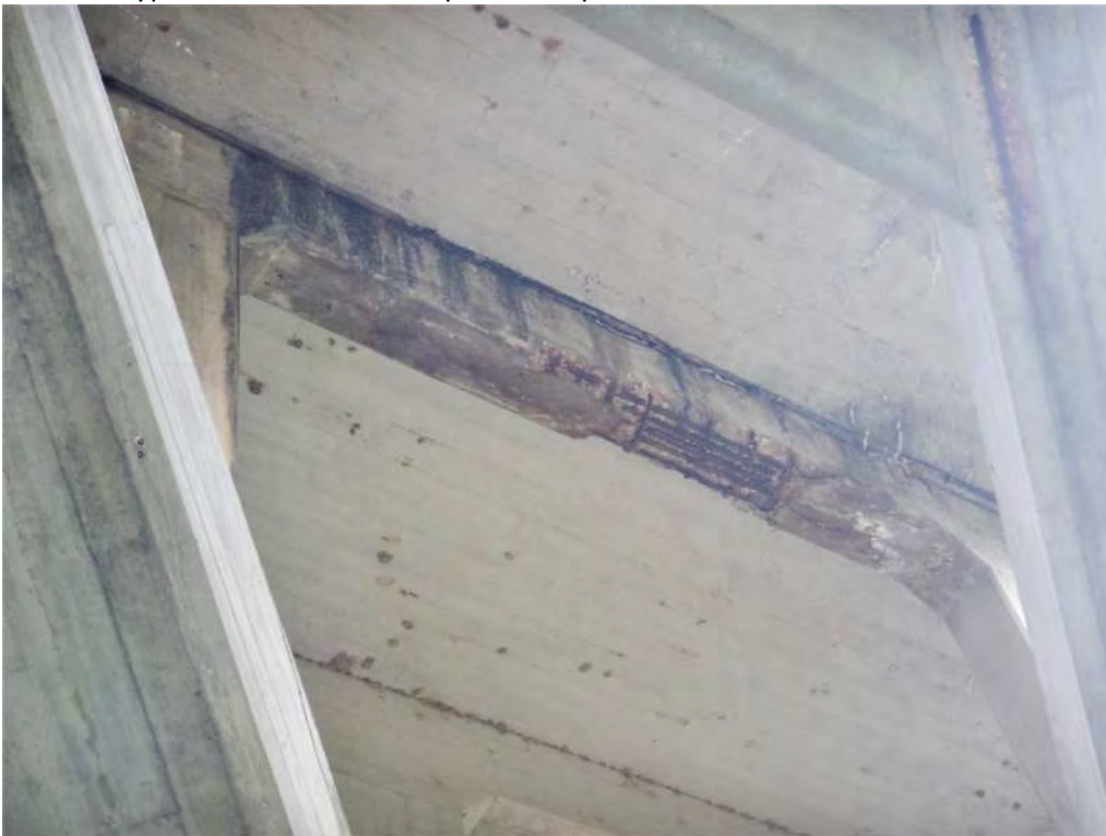
Pic. 006: Typical deterioration of spandrel capbeams
