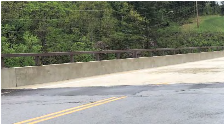
Figure 8-6. Vertical Concrete Barrier and Steel Tube Rail – Back Face
