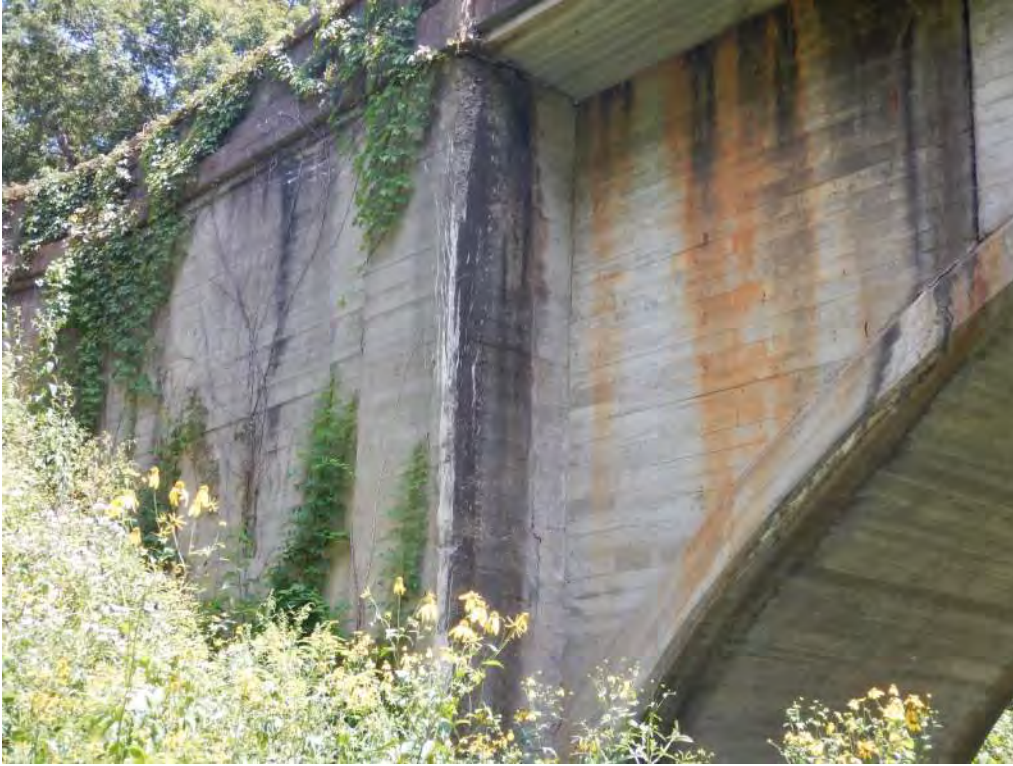
Pic. 007: Cracking and delamination, Abutment 1 west side
