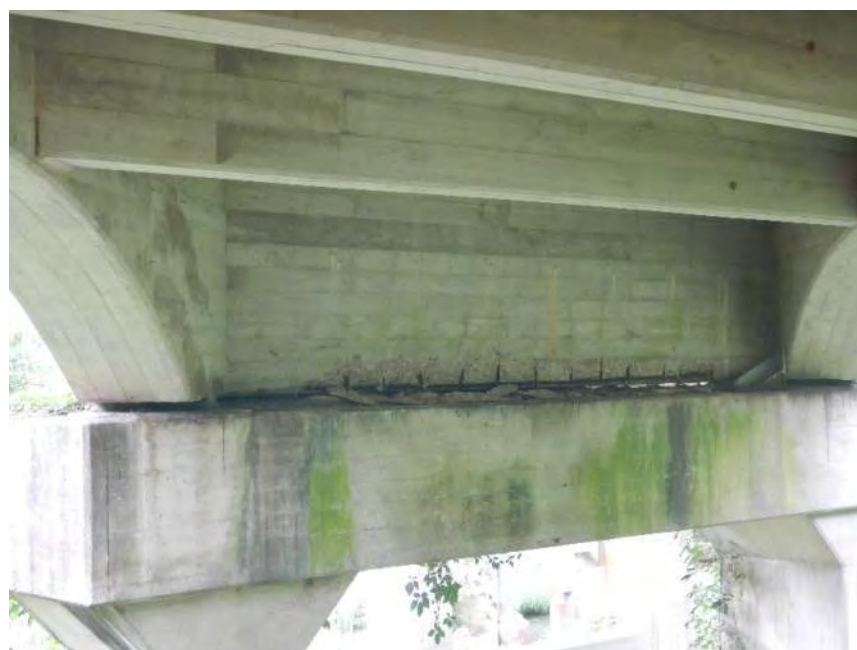
Deterioration of Floorbeams at Intermediate Bents
