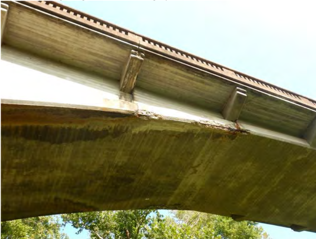
Pic. 005: Spalling along corner of arch ring, Span (4-5) east face
