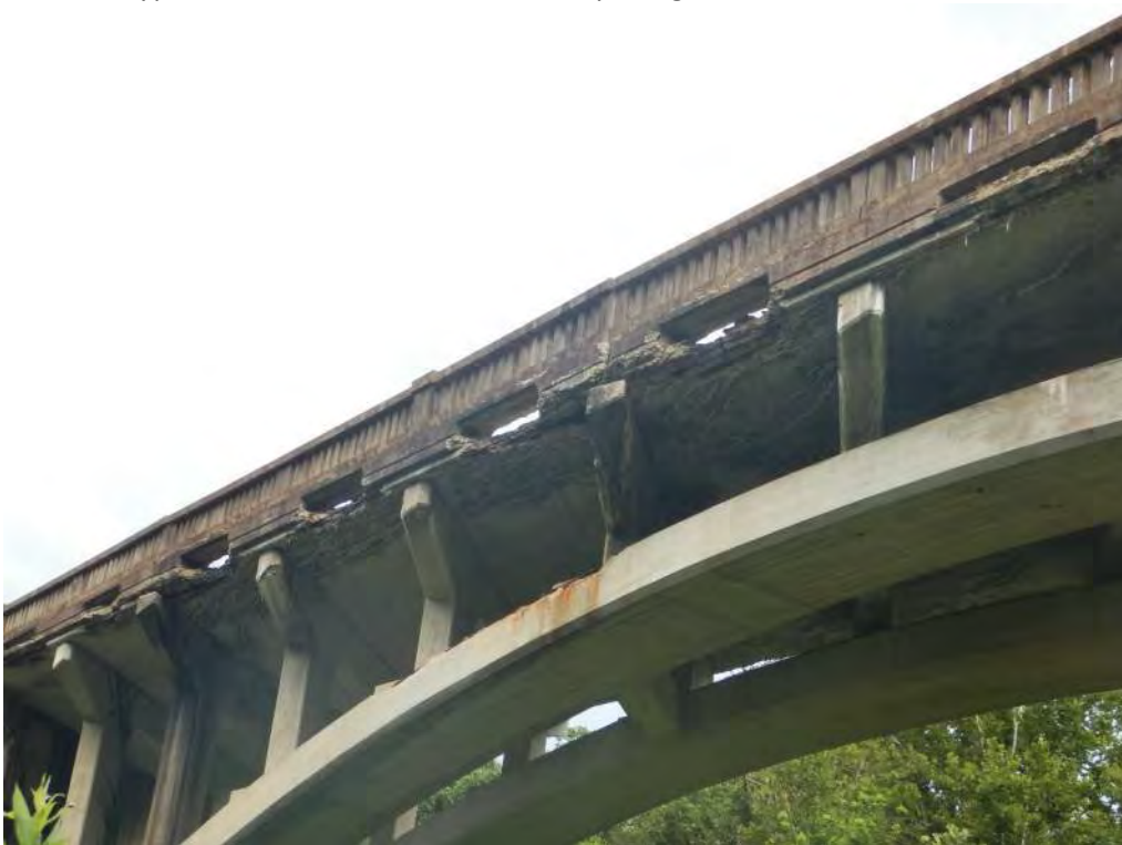
Pic. 002: Typical deck condition below curb openings
