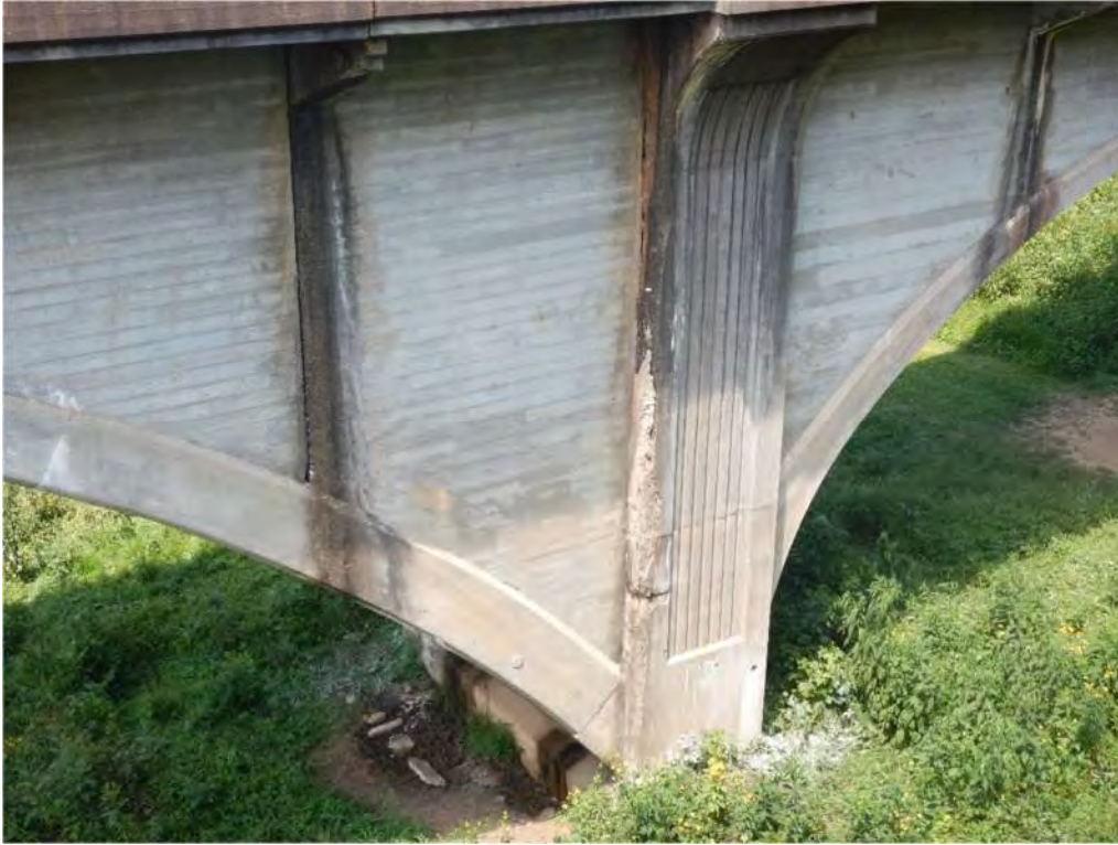
Pic. 009: Spalling and delamination on pilaster, Pier 2 east side
