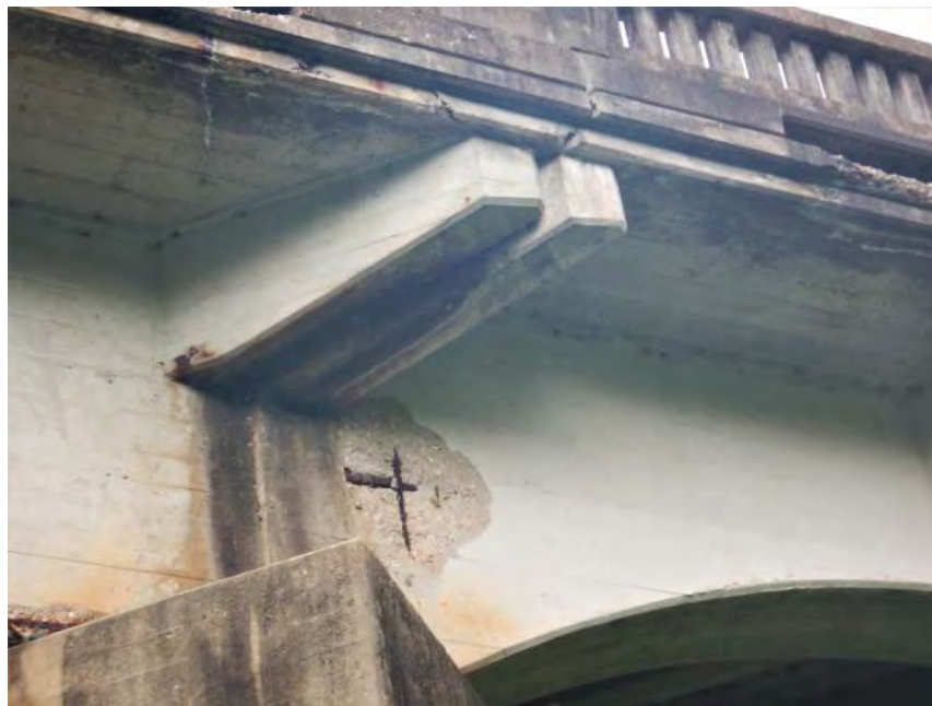
Typical Delamination on Girders
