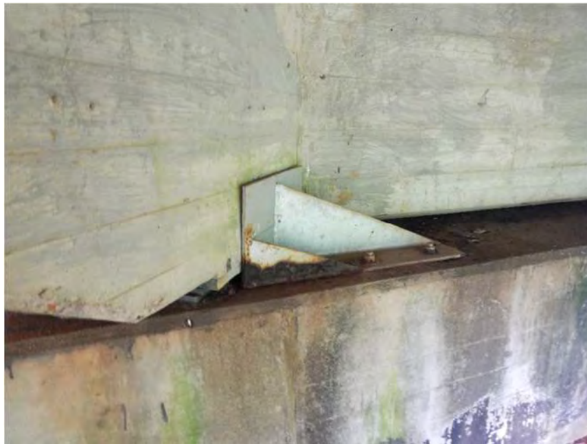
Typical Girder Restraint Bracket
