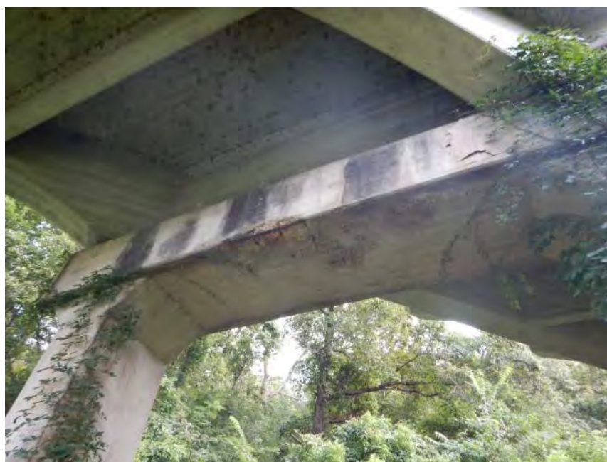
Deterioration of Intermediate Bent Cap Beams
