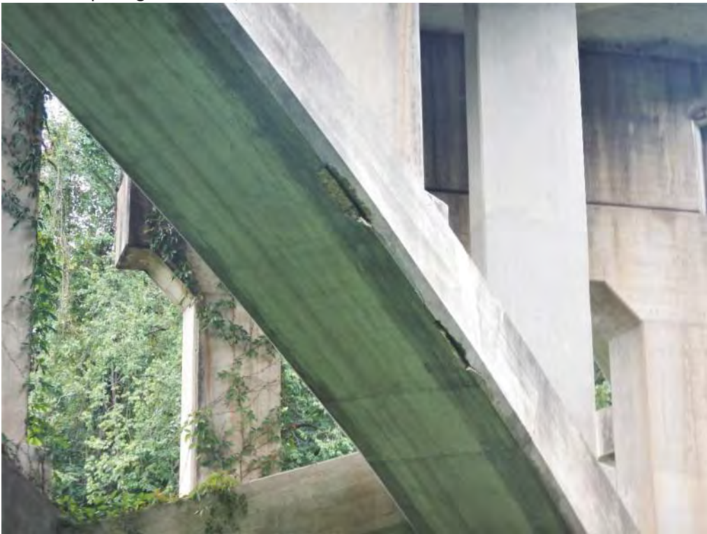
Pic. 008: Spalling of arch rib, west rib near south thrust block
