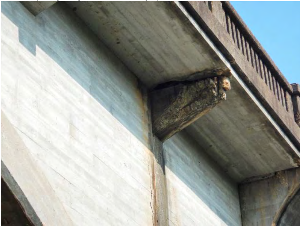
Pic. 006: Spalling along corner of arch ring, Span (4-5) east face
