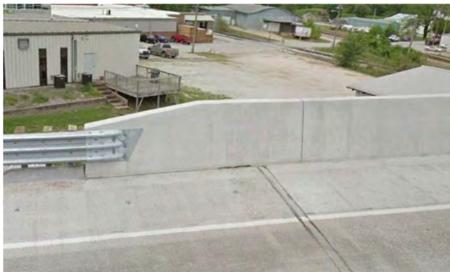
Figure 8-4. MoDOT Type D Concrete Barrier Curb
