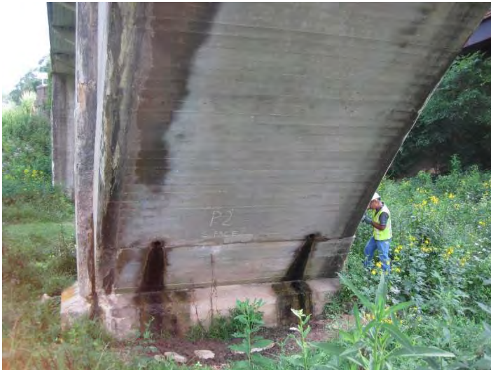
Photo 4: CRB, Typical leakage from drains at base of arch
