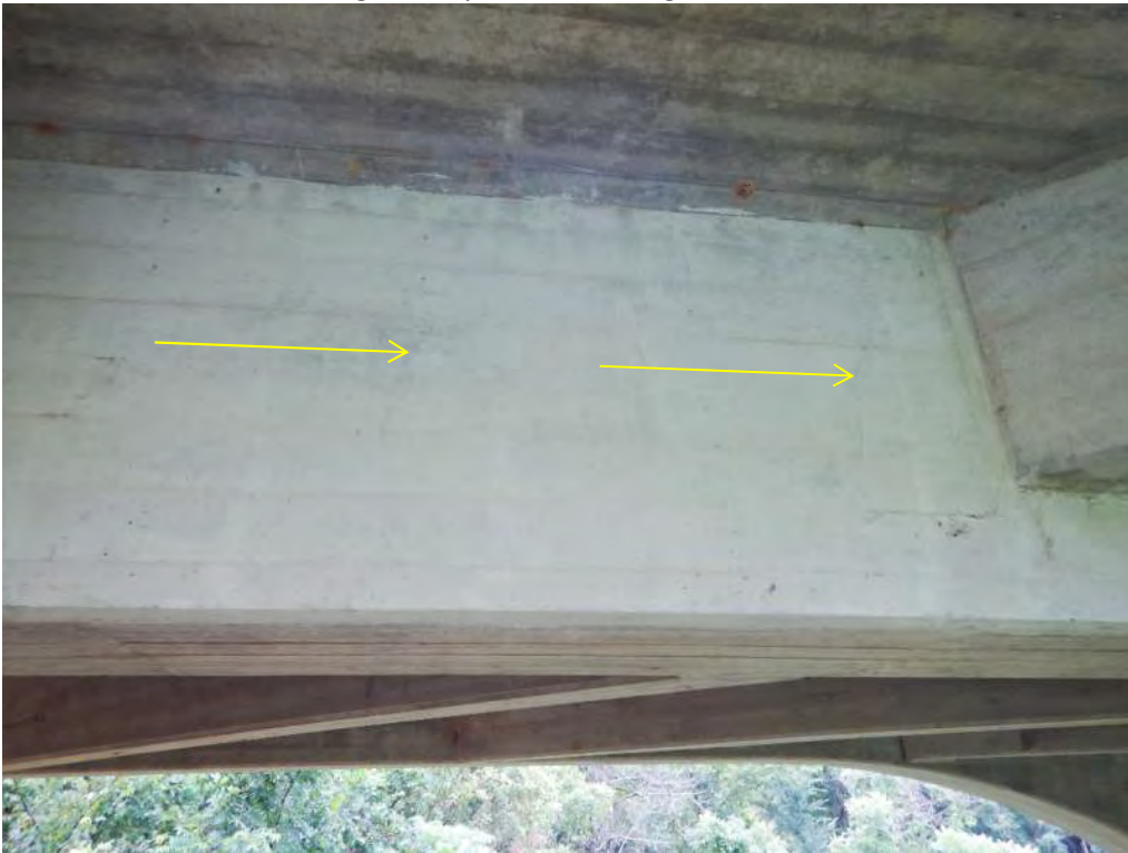
Pic. 004: Hairline cracks in girder, Span )1-2) west girder shown
