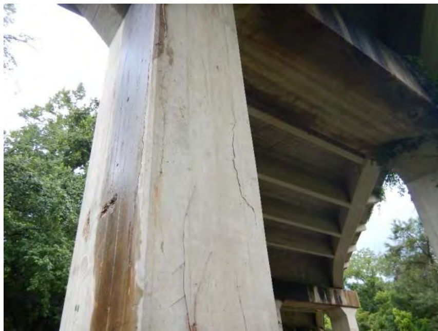
Deterioration of Intermediate Bent Columns
