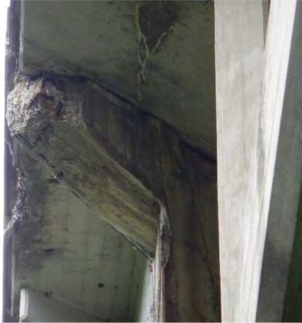
Typical Deterioration of Brackets
