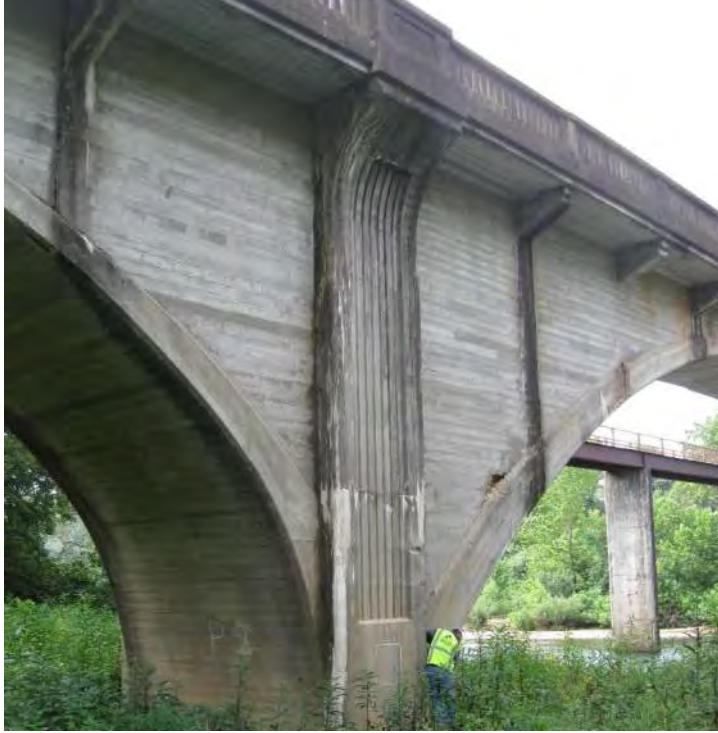
Photo 3: CRB, Typical Leakage from vertical joints in fascia walls
