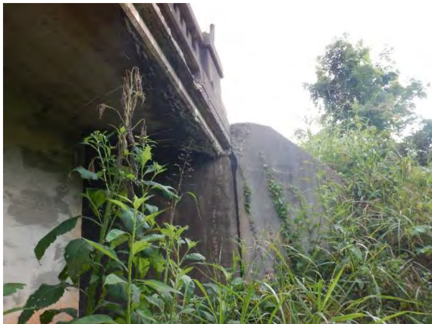
Typical Spalling at Abutment
