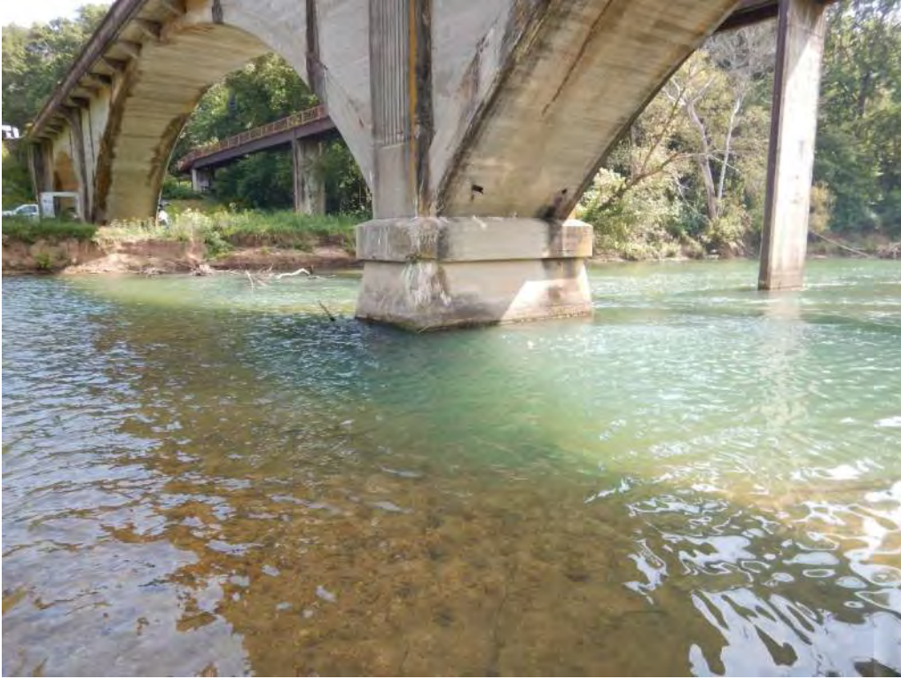
Pic. 011: Scour hole at Pier 3
