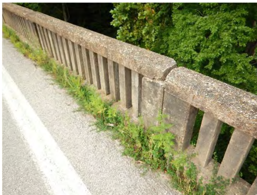
Collision Damage to the Railing
