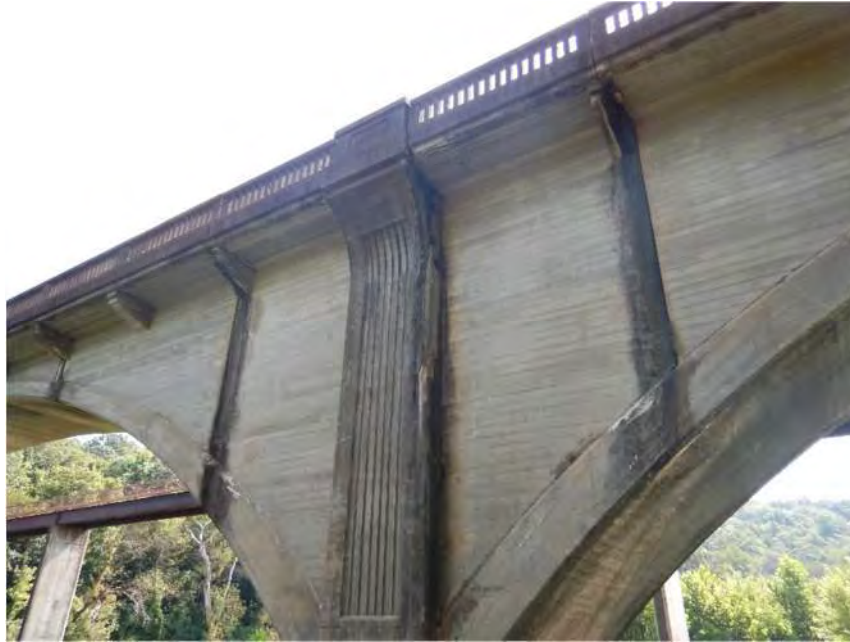
Leakage from Sidewall Joints
