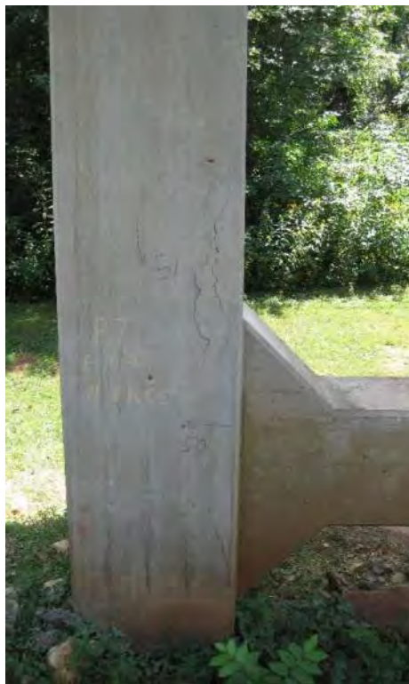
Photo 6: SVB, Typical Cracking and exposed reinforcement, Pier 7, North Face, east column and Pier 6, East Face, east column shown
