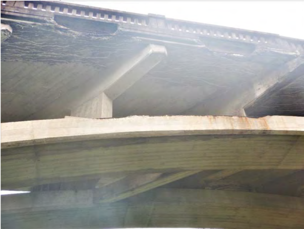
Pic. 007: Spalling near center of arch rib, east rib
