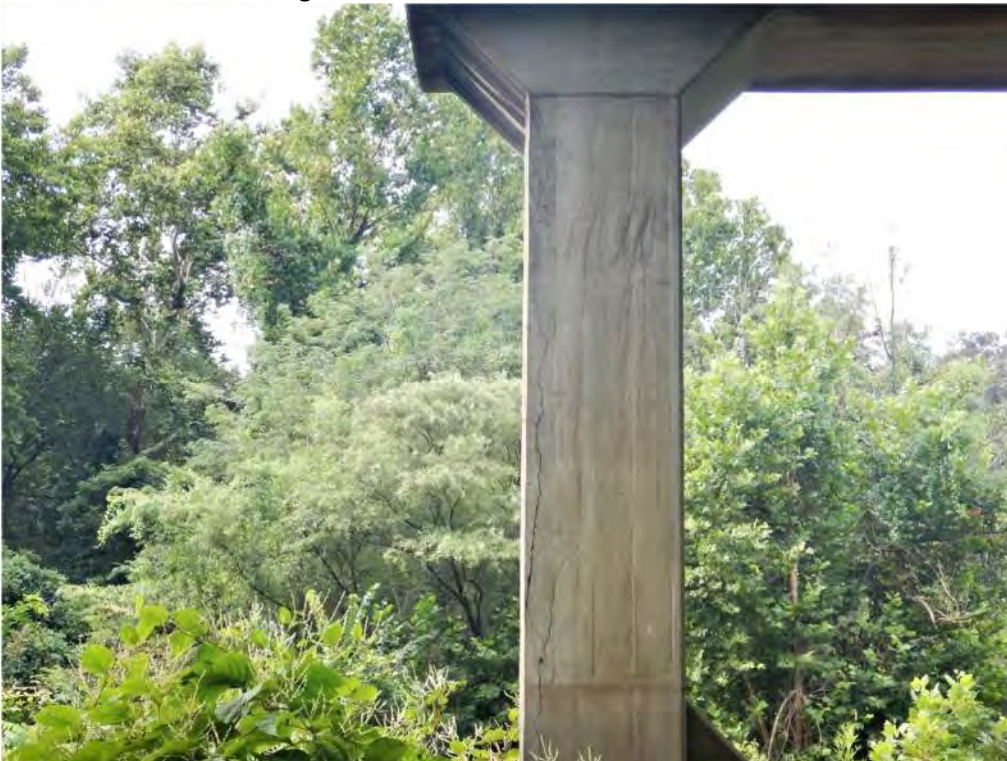
Pic. 010: Vertical cracking in column, Bent 3 shown
