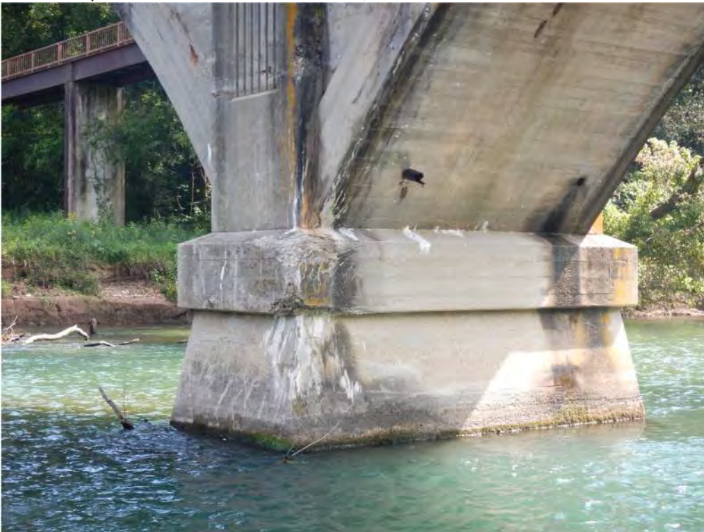
Pic. 008: Spalled and deteriorated concrete, Pier 3 west face
