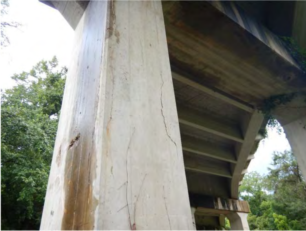
Pic. 011: Spalling and cracking on column, Bent 6 shown
