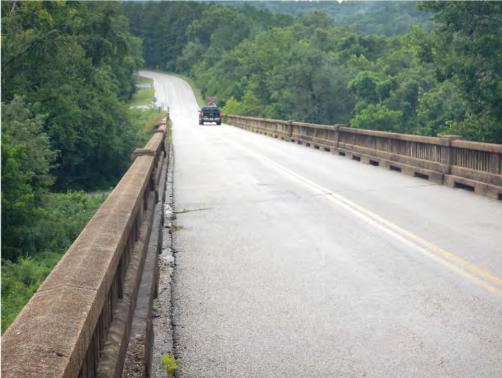
Pic. 003: Bridge barrier rail with misalignment
