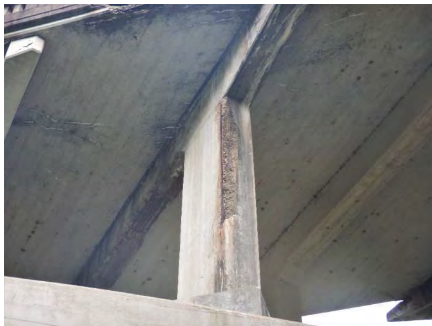
Typical Deterioration on Spandrel Columns
