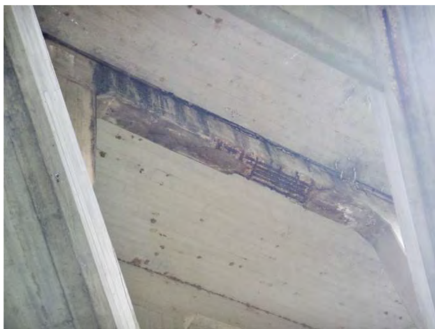
Typical Deterioration on Spandrel Capbeams
