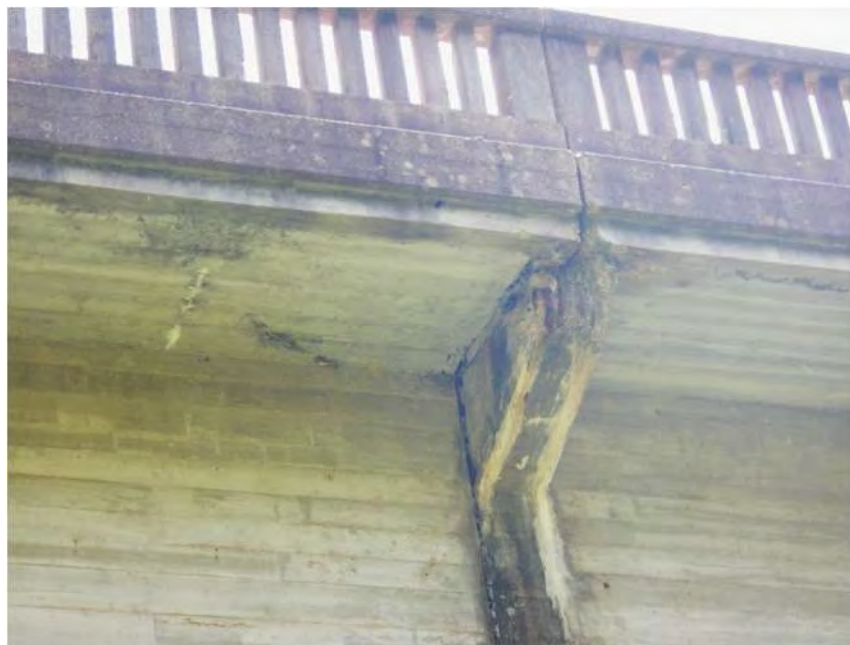
Heavy Deterioration with Loss of Bracket Support Area
