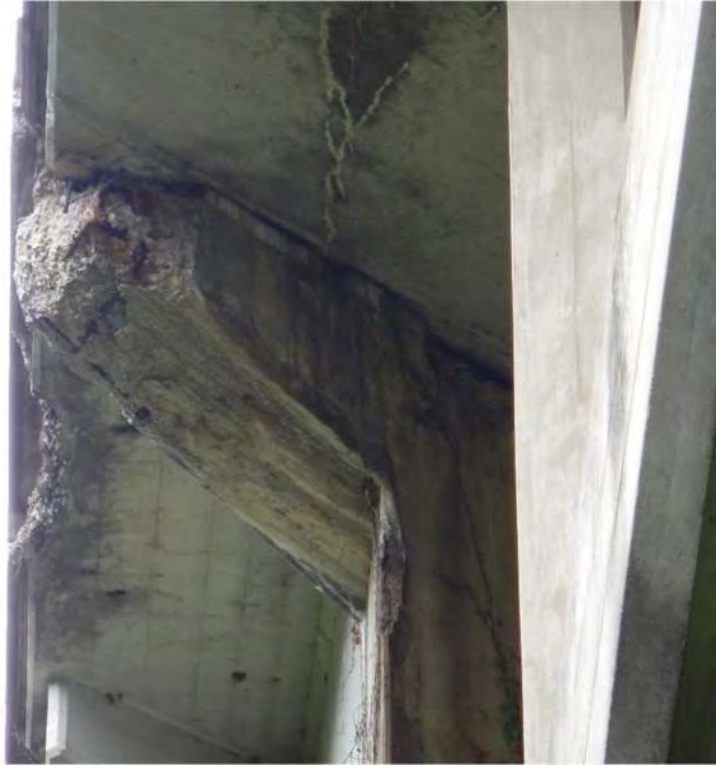
Pic. 005: Deterioration of cap beam cantilever
