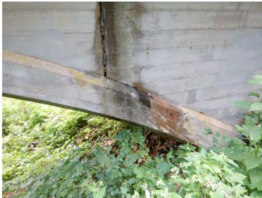
Spalling and Staining on Arch Ring
