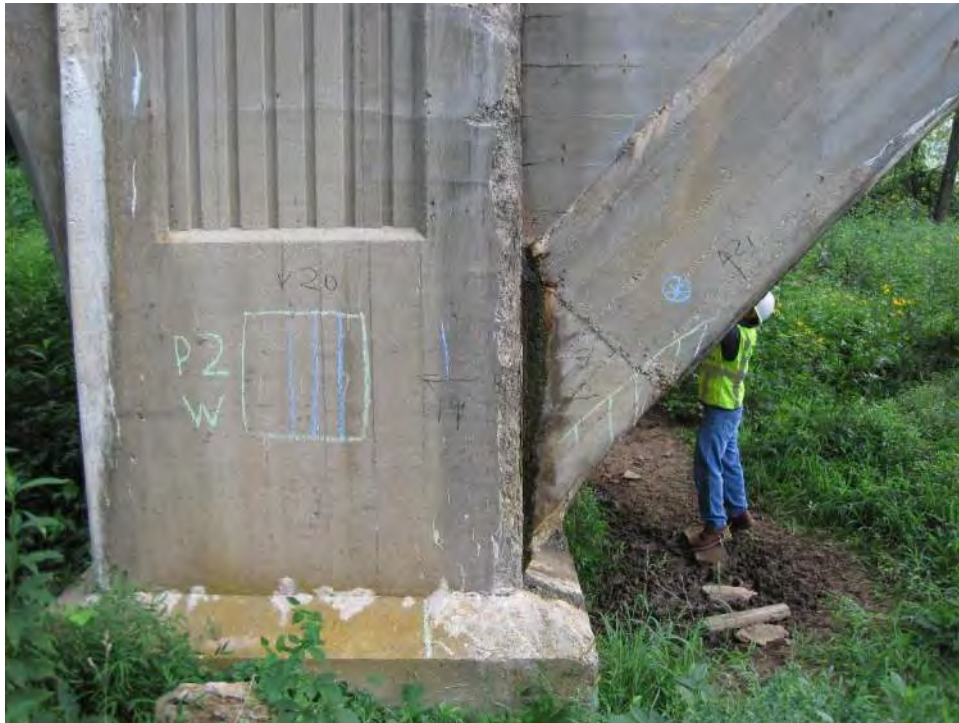
Photo 2: CRB, Typical spalling and deterioration along vertical corners of pier and edge of arch, West Face, pier 2 shown.
