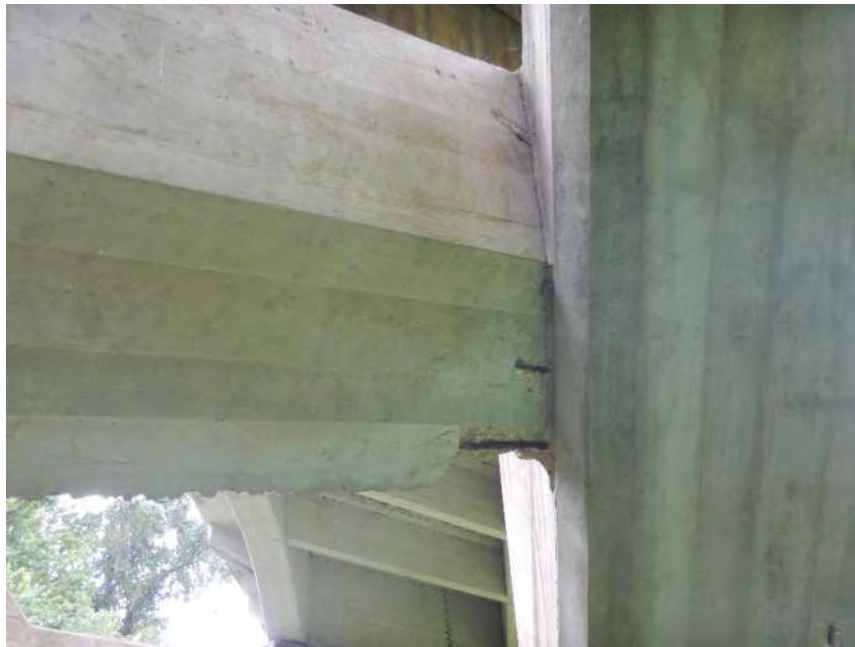
Lateral Bracing Between the Arch Ribs
