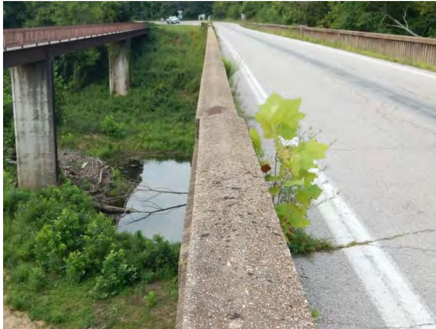
Differential Alignment of Barrier at Joints Adjacent to Pier
