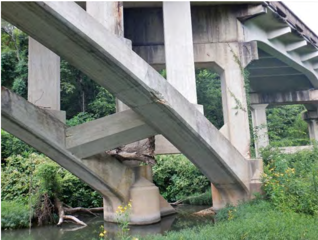
Pic. 012: Scour hole at Pier 4
