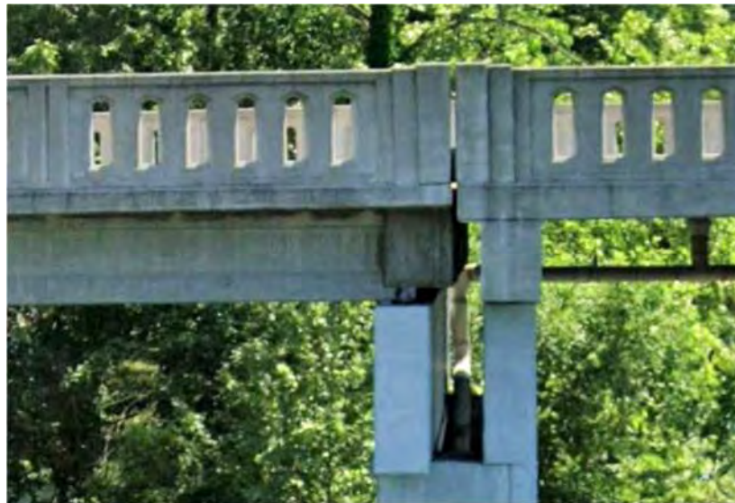
Figure 8-9. Open Concrete Curb and Rail with Concrete Posts – Back Face
