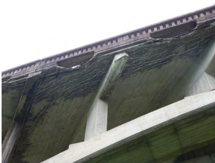
Heavy Deterioration of the Deck at Existing Drains
