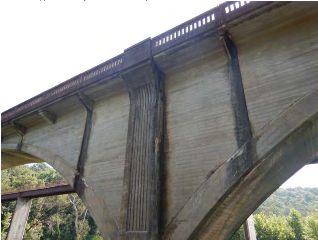
Pic. 002: Typical leakage from sidewall joints
