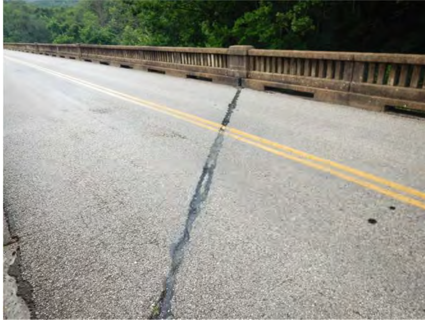
Typical Slab Expansion Joint
