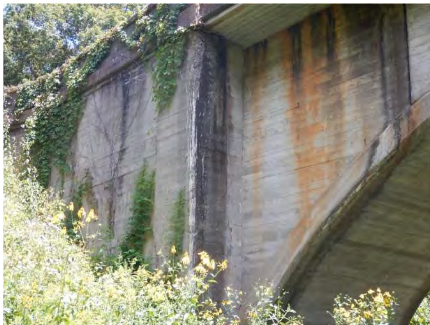
Cracking and Delamination at Abutments
