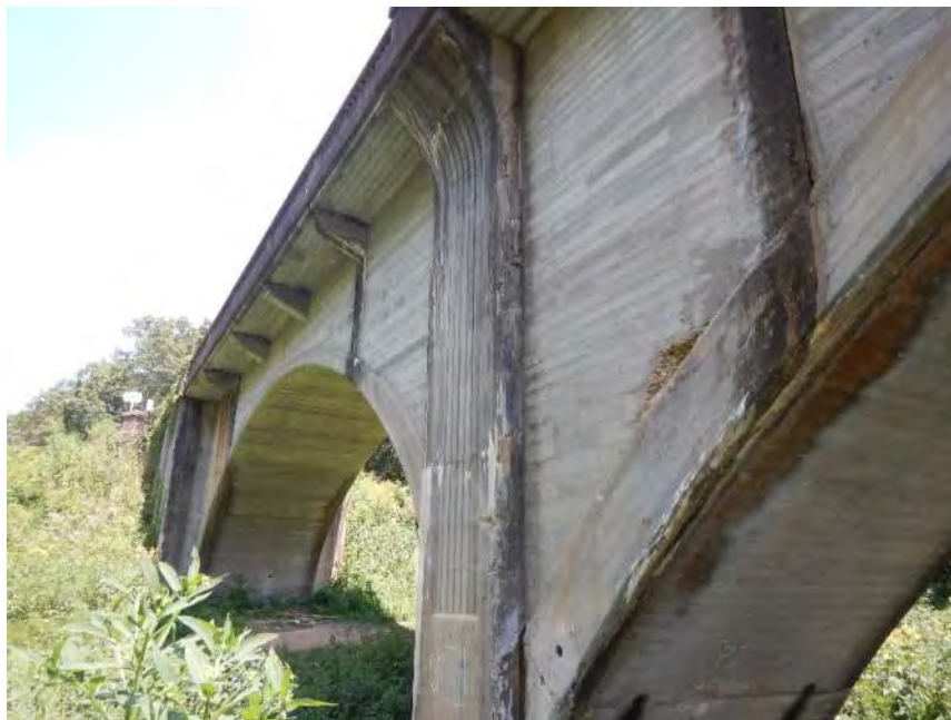
Spalling on Pier Surfaces
