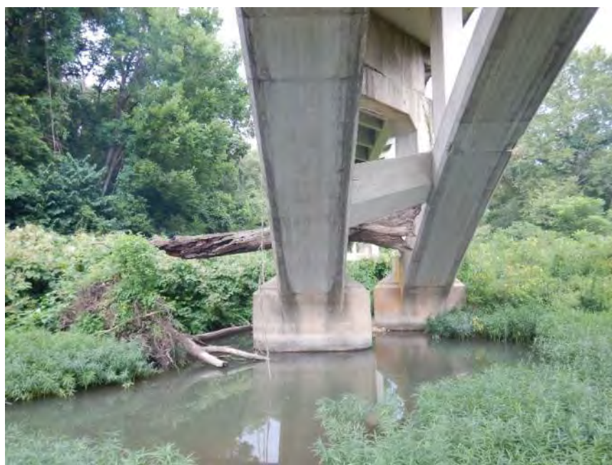
Drift in Structure
