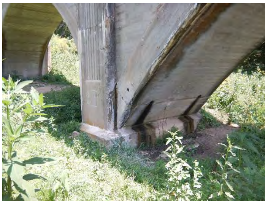
Scaling Along Pier Foundations
