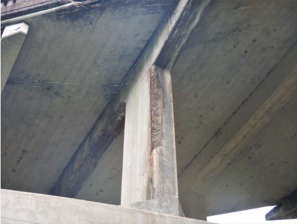
Pic. 009: Typical deterioration of spandrel column
