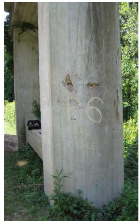
Photo 6: SVB, Typical Cracking and exposed reinforcement, Pier 7, North Face, east column and Pier 6, East Face, east column shown
