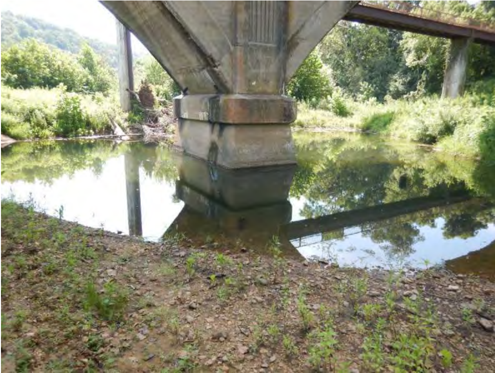
Pic. 012: Scour hole at Pier 4
