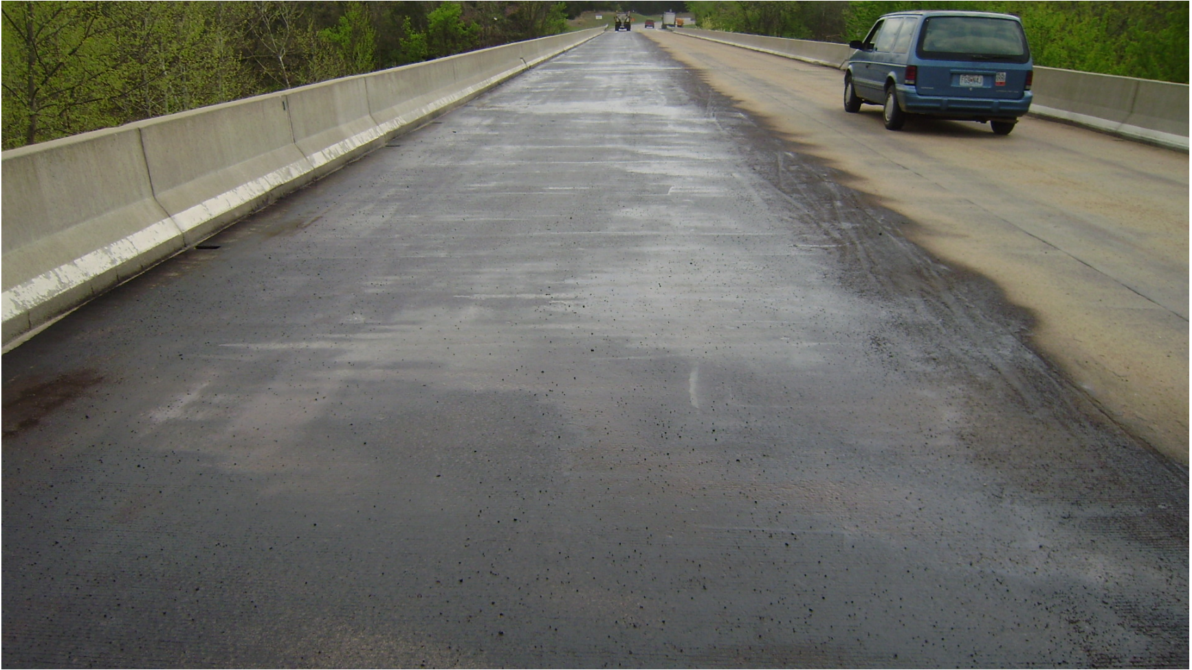
Typical bridge deck seal
