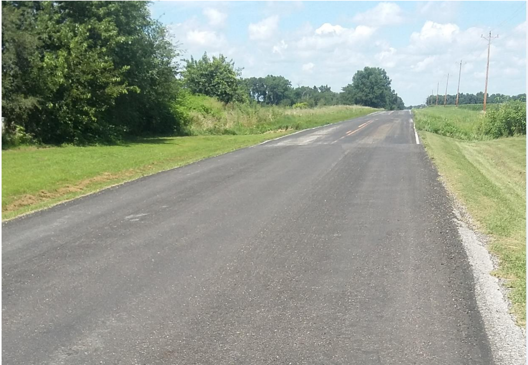
Typical asphalt pavement repair
