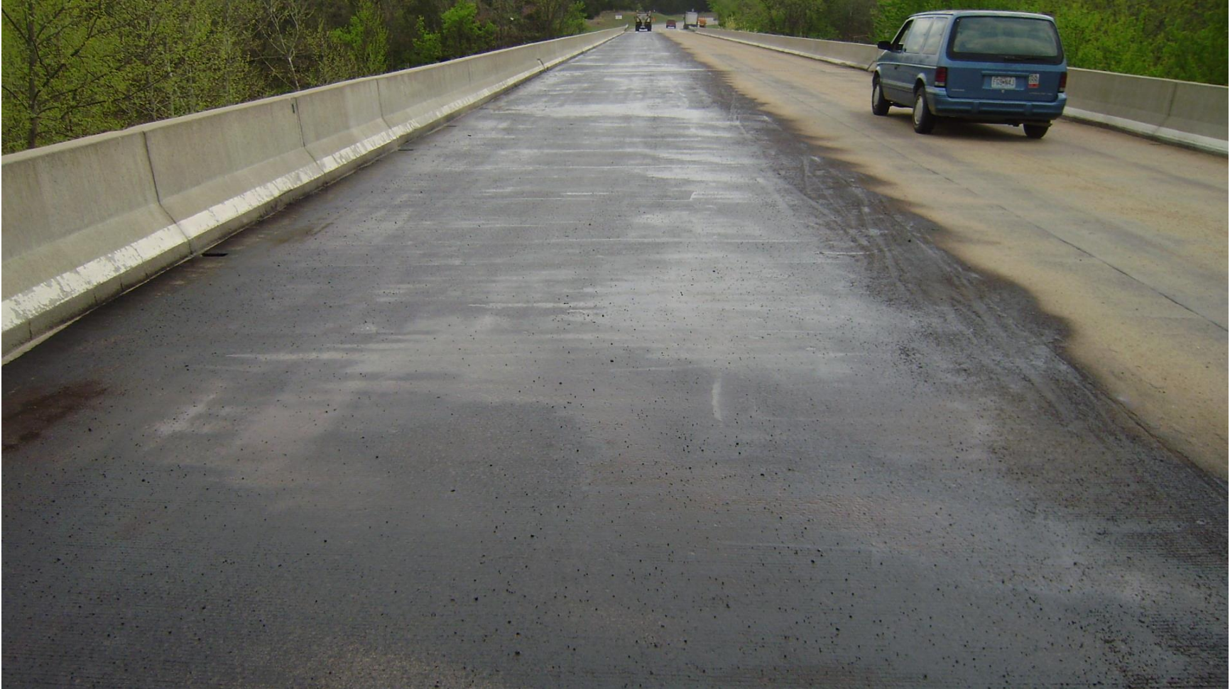
Typical bridge deck seal
