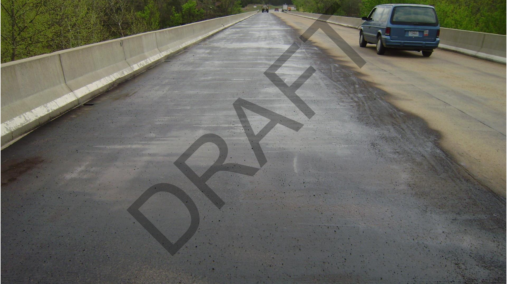
Typical bridge deck seal
