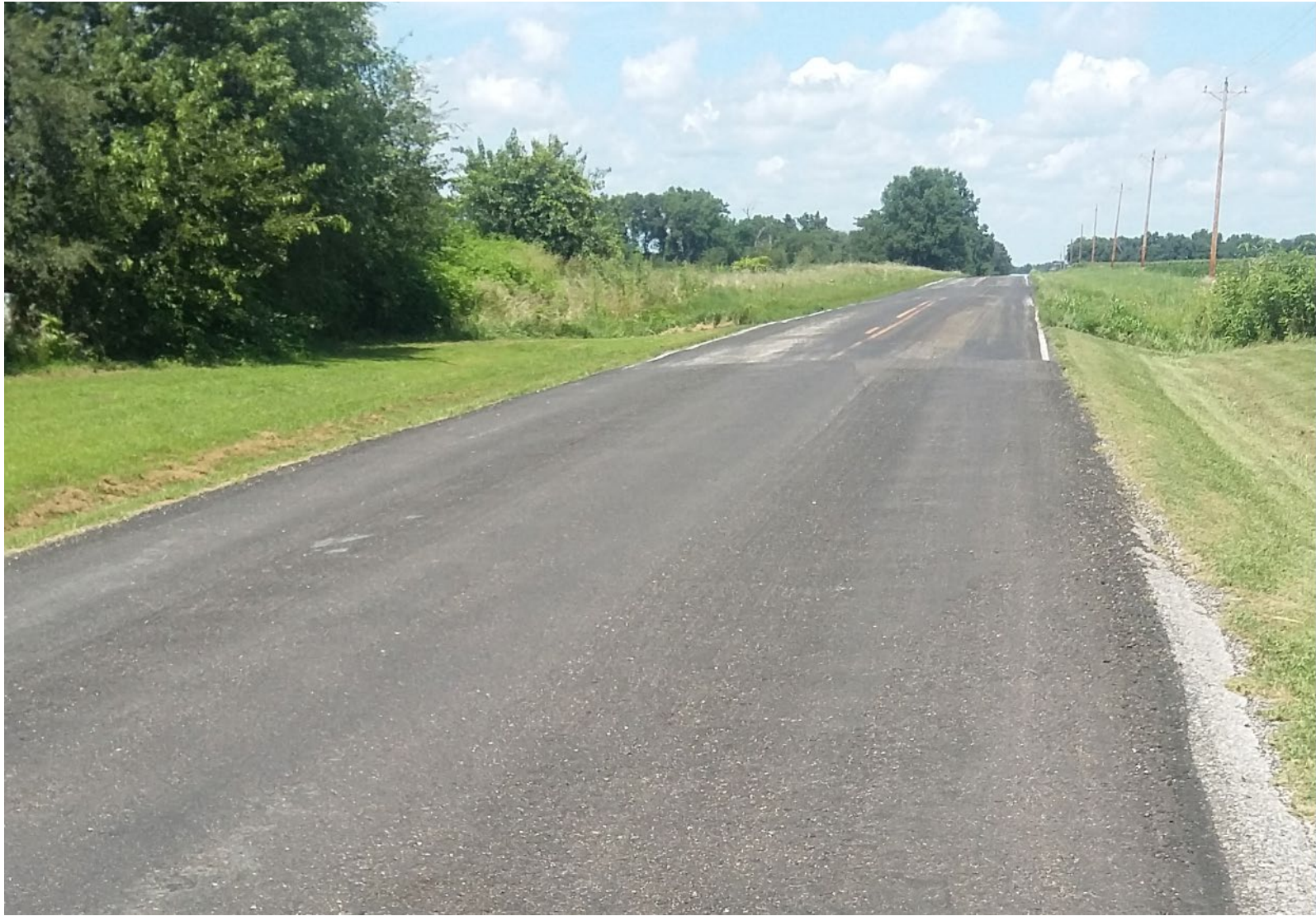
Typical asphalt pavement repair
