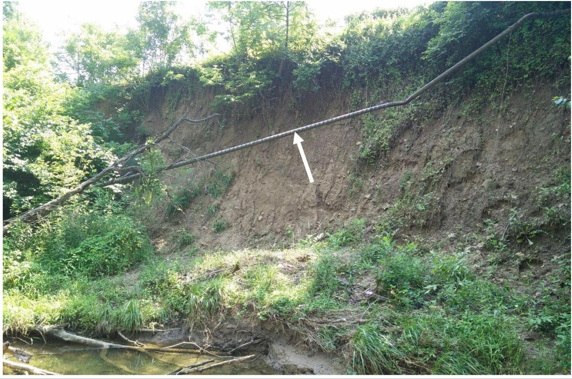
**Creek Bank E is steeply sloped to vertical with exposed utility line. (facing Southeast at the creek bend)**
