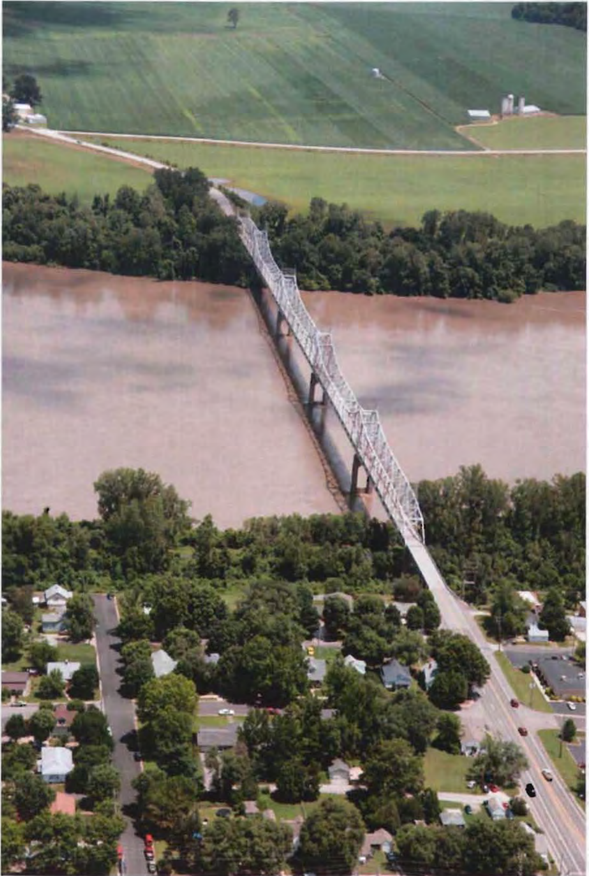
Washington Bridge (K0969). View to north.
