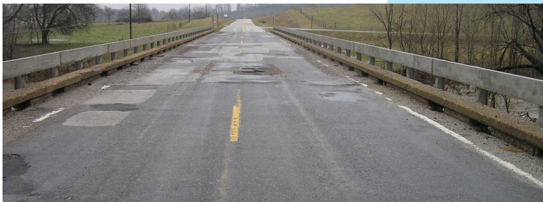
Existing Woods Fork Bridge
