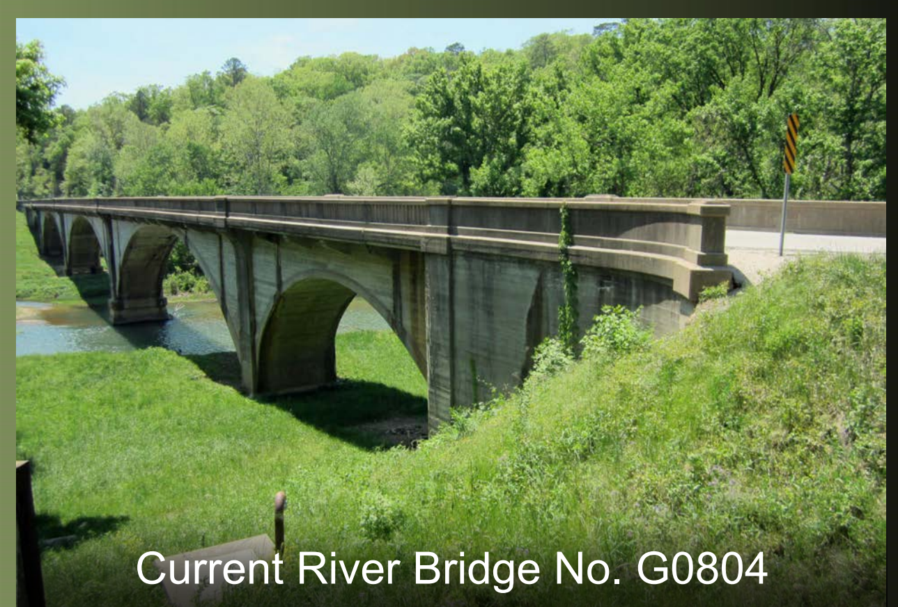
Current River Bridge No. G0804
