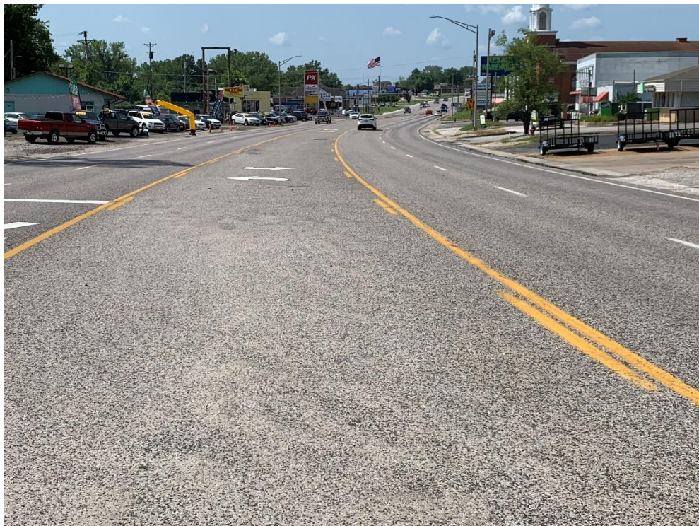
An example of a two-way left turn lane
