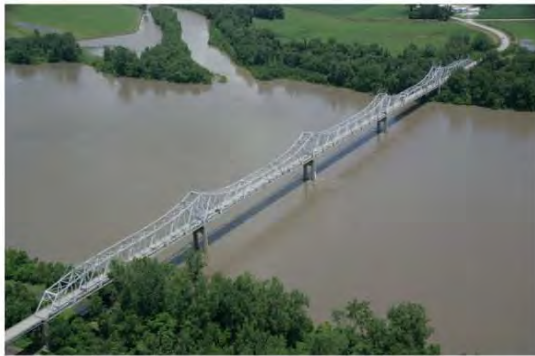
Route 47 Bridge from above, facing north
