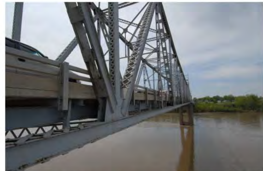
Side view of bridge showing lower chord and road deck
