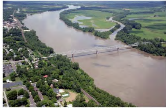
Aerial view of Route 47 Bridge, looking upstream
