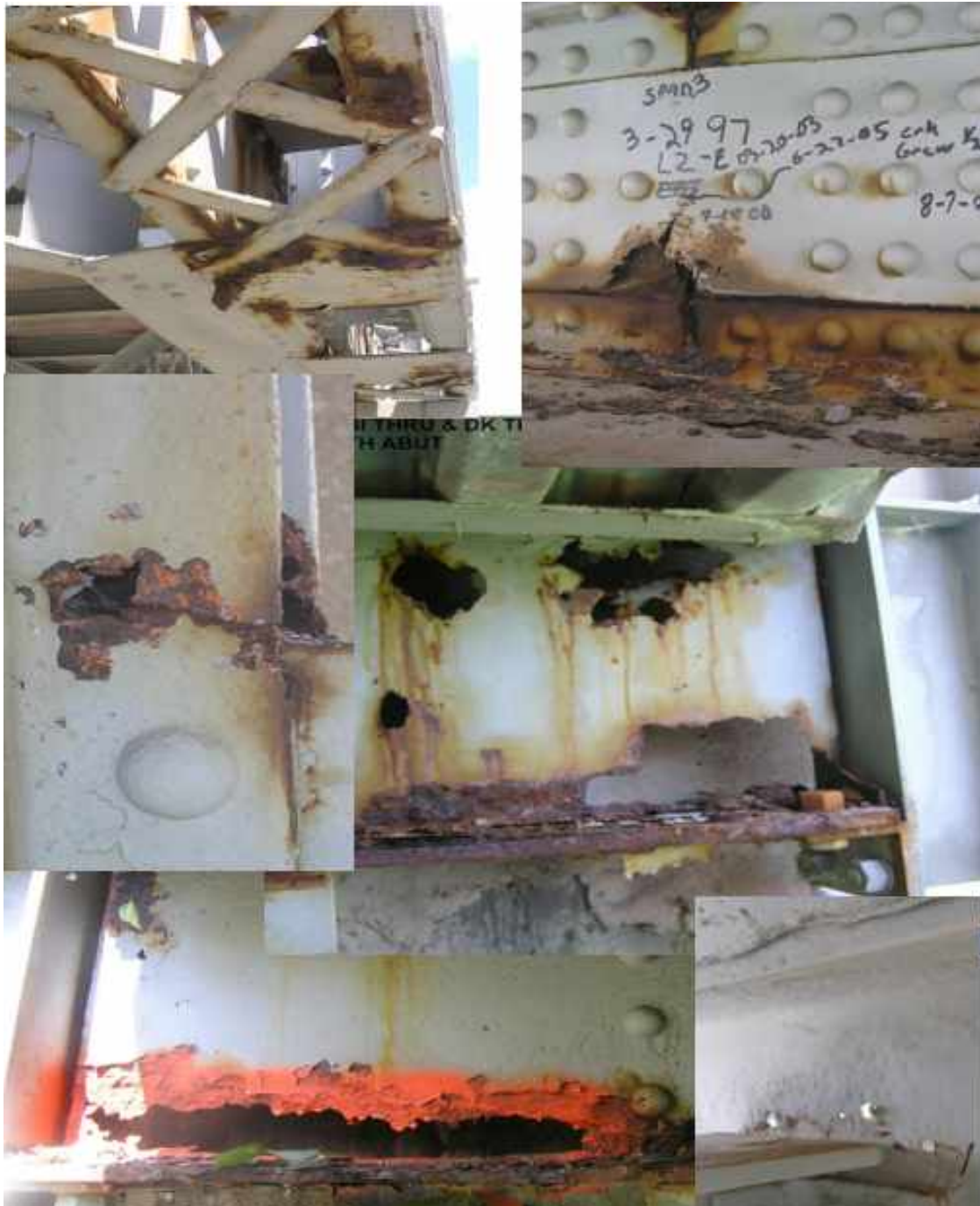
Figure 4. Photo Collage of Bridge Condition before 2009 Rehabilitation
