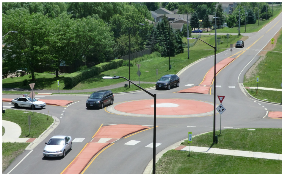
Example of a single-lane roundabout. Source: FHWA
