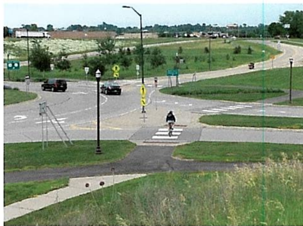
Example of a multi-lane roundabout.
