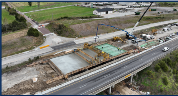
The bridge deck of the brand new direct connection flyover ramp from northbound U.S. 63 to westbound I-70 was poured in October 2026.
