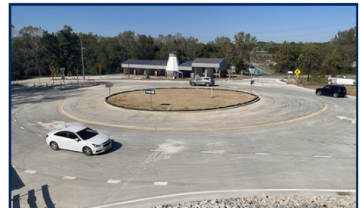
New Clark Lane roundabout has opened in Columbia.
