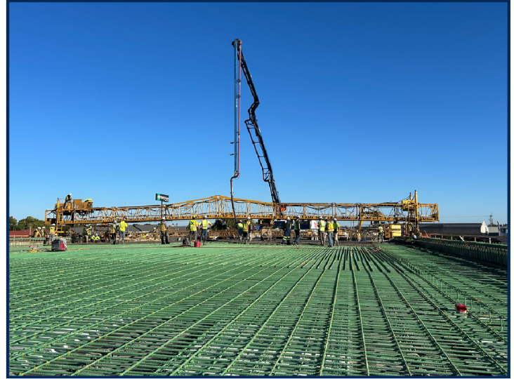
The bridge deck of the Providence Road bridge over I-70 was poured on October 6 in Columbia.
