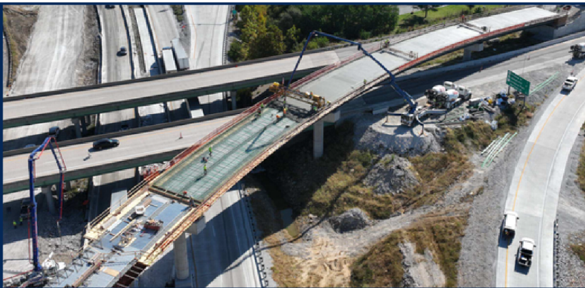
The bridge deck of the brand new direct connection flyover ramp from northbound U.S. 63 to westbound I-70 was poured in October 2026.
