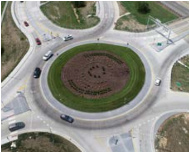
Lake Saint Louis Boulevard / I-70 Roundabout in Lake Saint Louis - This MoDOT LPA project converted the interchange to a 6-legged roundabout with new sidewalks, a retaining wall, and storm sewer modifications. The roundabout recently received the Project of the Year award by the American Public Works Association (APWA).
