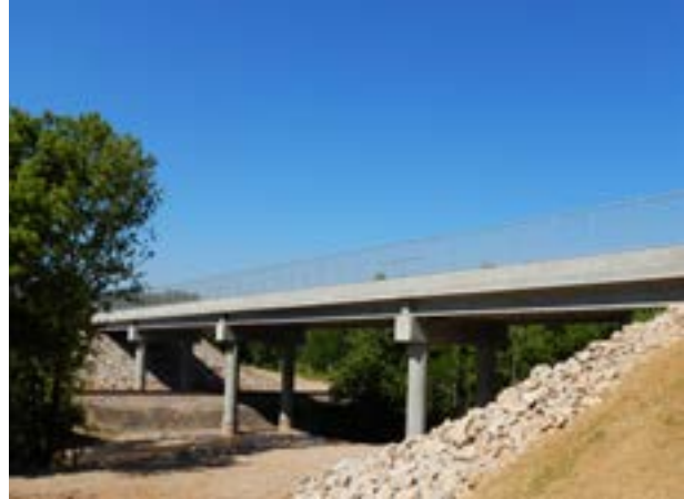
Replacement of an existing bridge in Sikeston, Missouri - Oates worked with MoDOT, SE district to replace the existing truss bridge and design a new 3-span steel bridge with pedestrian facilities at Business Route 63 over Two Mile Creek and BNSF Railroad.
