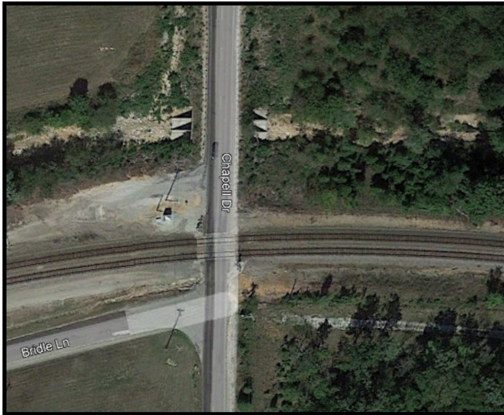
2. Image of Existing RCB Crossing over Kelly Creek
