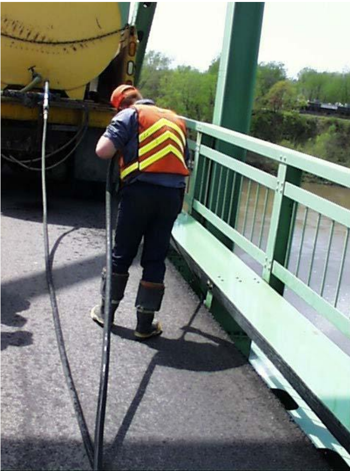
Adequate water supply and pressure is needed for effective flushing.
