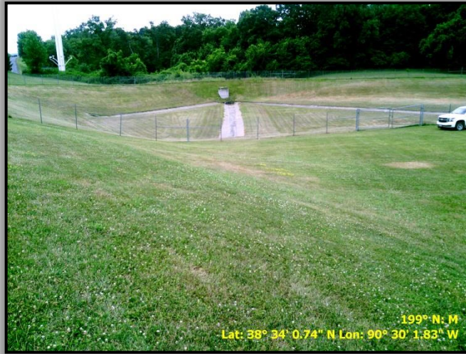
Figure 1: Permanent detention basin on Route 141 and Big Bend Rd.
