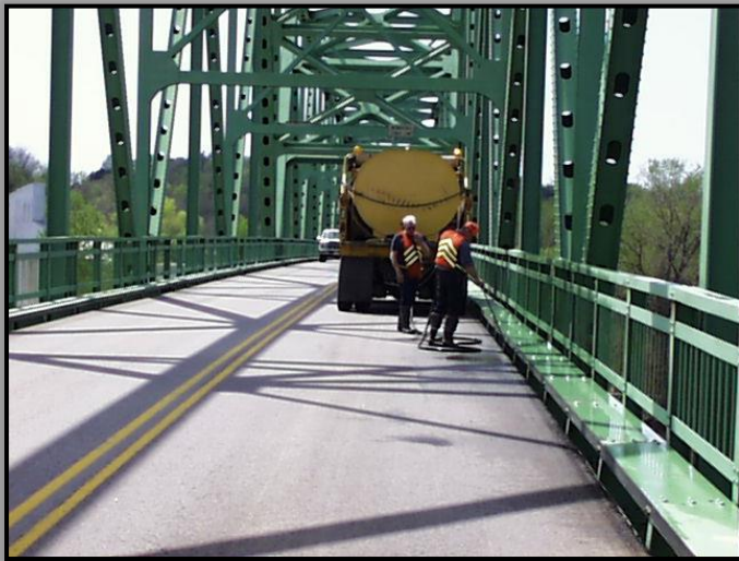
Figure 1: Street sweeping and bridge washing.
