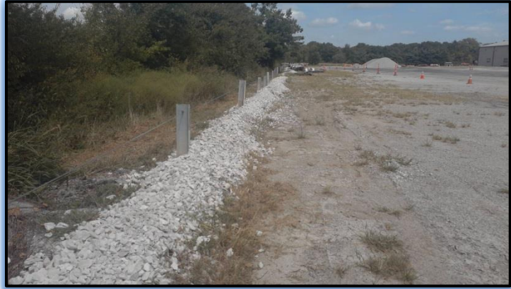
Figure 4: Maintenance facility in SW District.
