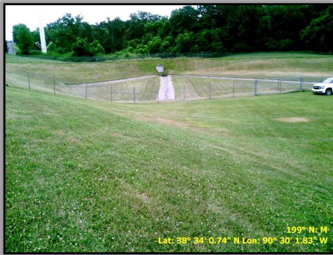
Figure 2: Permanent detention basin on Route 141 and Big Bend Rd.
