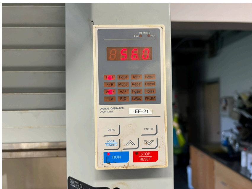
Figure 4: Lab Exhaust Controller Mounted on Hood
