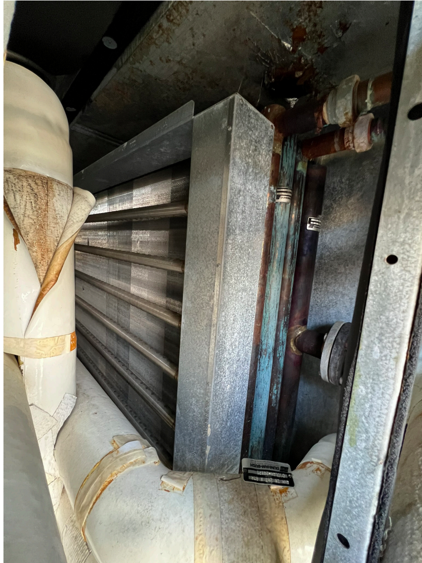
Figure 8: Preheat, Cooling, and Reheat Stacked in an Air Handler
