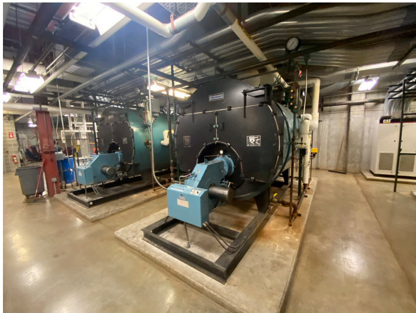
Figure 1: Existing Steam Boilers
