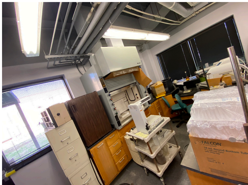
Figure 13: Example of Auxillary Hood Supply Being Blanked Off
