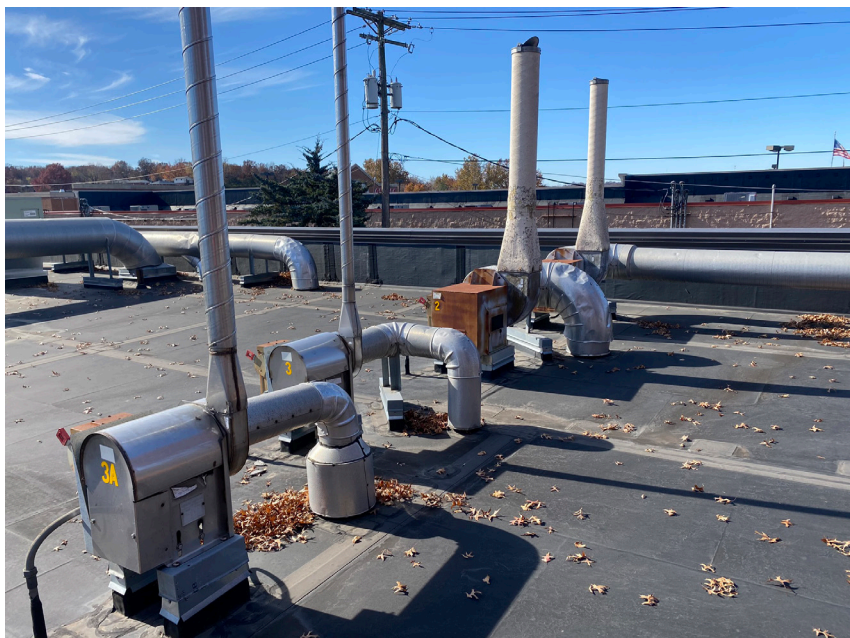
Figure 10: Exhaust Fans Above Instrumentation Lab
