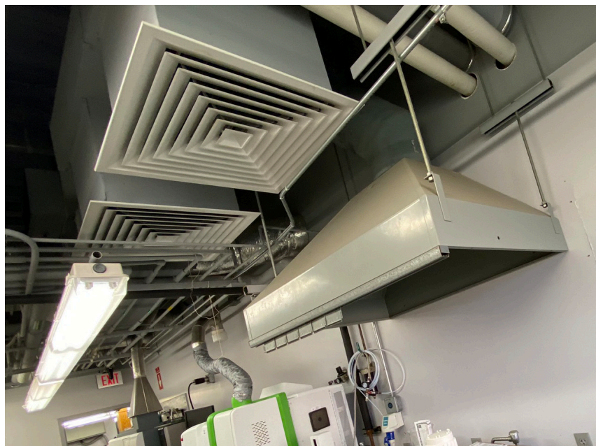
Figure 12: Example of Four Way Diffusers Placed Poorly
