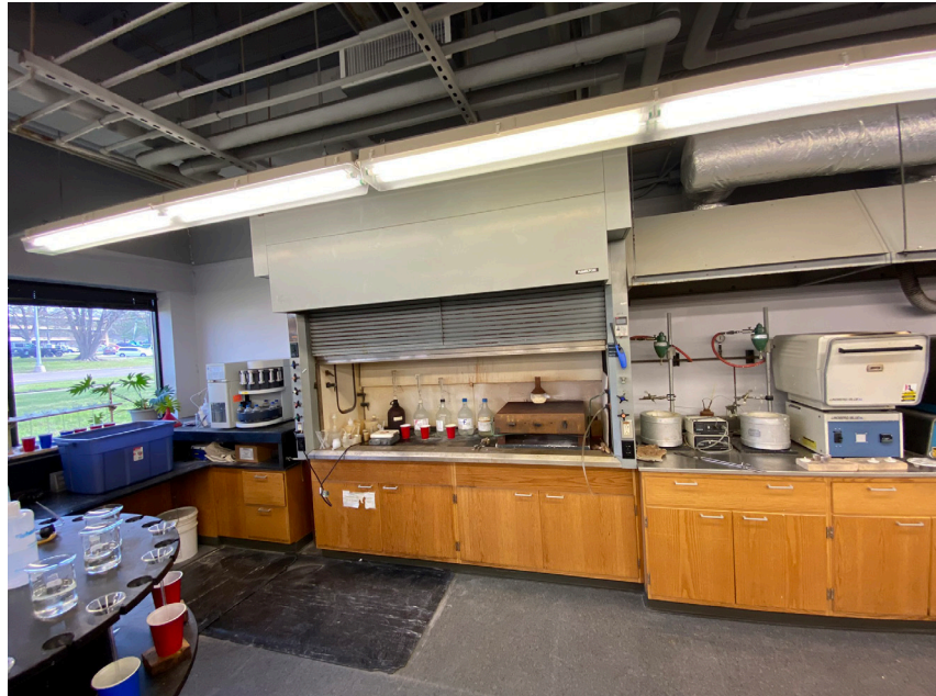
Figure 11: Laboratory Hood #9 with Example of Poor Air Distribution Device Above
