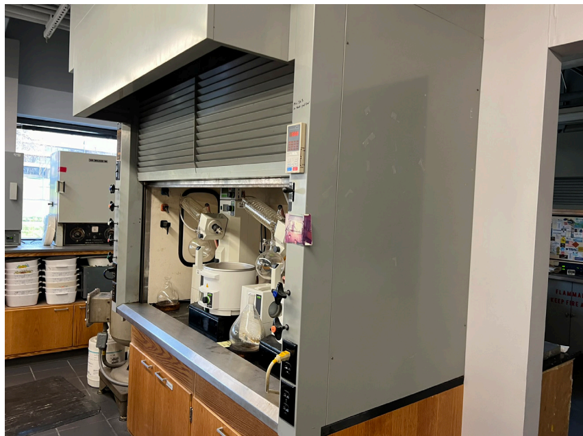
Figure 3: Typical Laboratory Exhaust Hood
