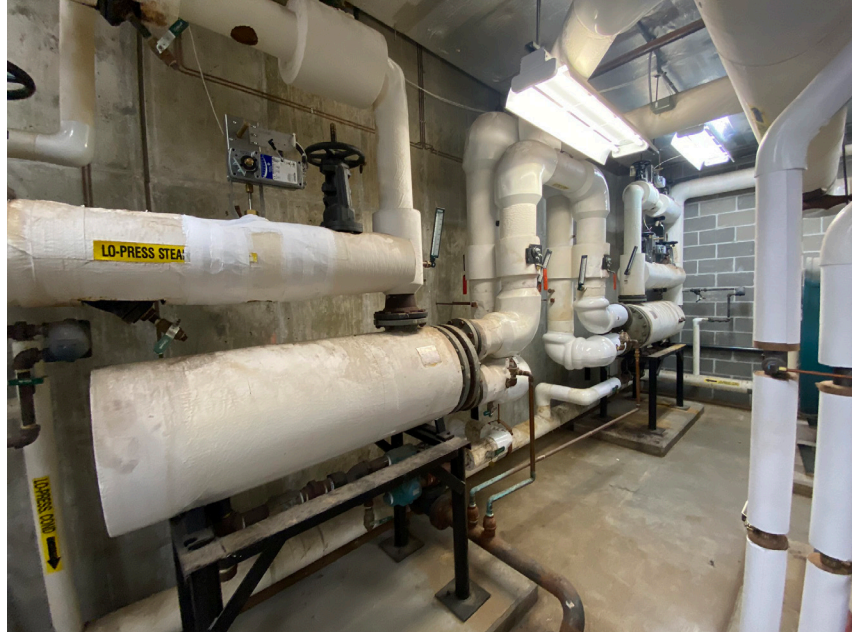
Figure 2: Shell and Tube Steam to Hot Water Heat Exchangers
