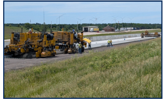
Paving progress in Lafayette County.
