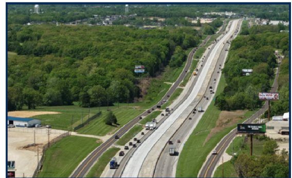
Paving progress in Warren County.
