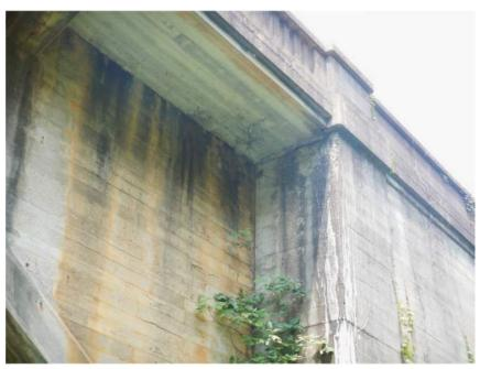
Typical Spalling at Abutment Corners
