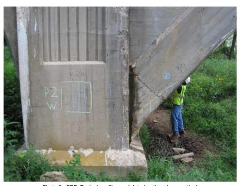
Photo 2: CRB, Typical spalling and deterioration along vertical corners of pier and edge of arch, West Face, pier 2 shown.
