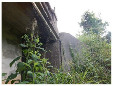
Typical Spalling at Abutment
