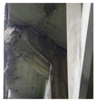
Typical Deterioration of Brackets
