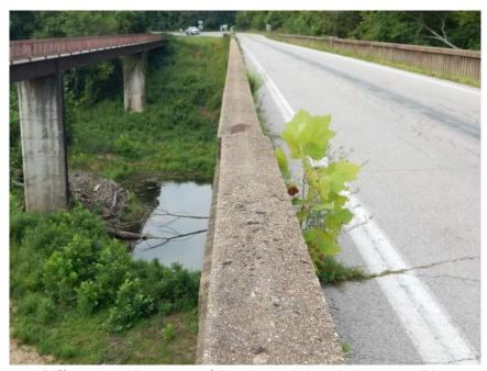
Differential Alignment of Barrier at Joints Adjacent to Pier
