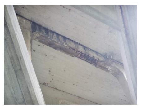
Typical Deterioration on Spandrel Capbeams
