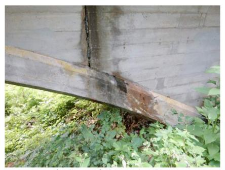
Spalling and Staining on Arch Ring
