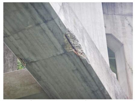
Spalling and Delamination of Arch Ribs
