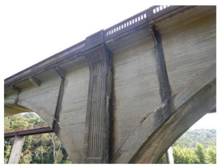
Leakage from Sidewall Joints
