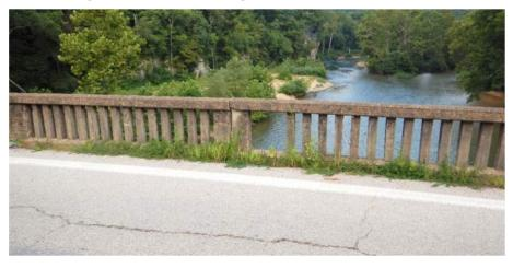
Figure 8-2. Existing Current River Bridge Rail – Back Face with Post
