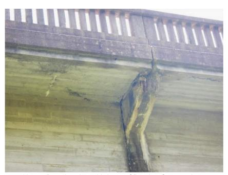
Heavy Deterioration with Loss of Bracket Support Area
