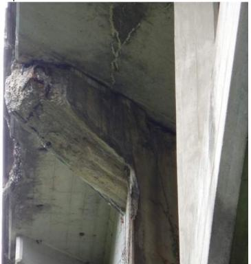
Pic. 006: Typical deterioration of spandrel capbeams
