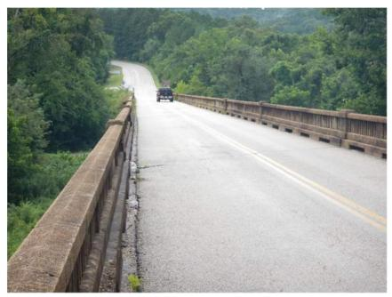
Collision Damage to the Railing
