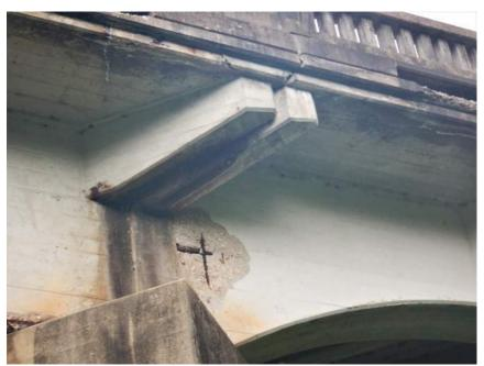
Typical Delamination on Girders
