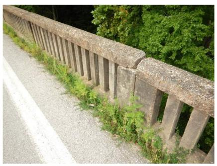
Collision Damage to the Railing
