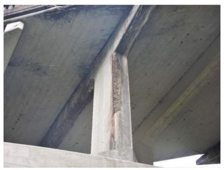
Typical Deterioration on Spandrel Columns
