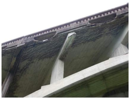
Heavy Deterioration of the Deck at Existing Drains
