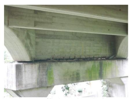
Deterioration of Floorbeams at Intermediate Bents
