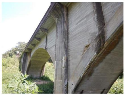
Spalling on Pier Surfaces
