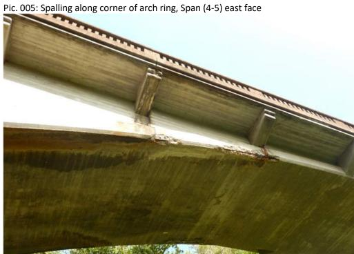
Pic. 006: Spalling along corner of arch ring, Span (4-5) east face
