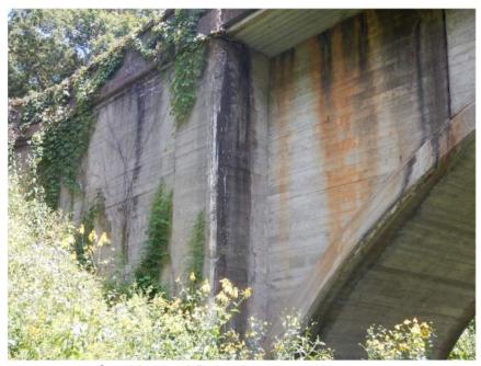
Cracking and Delamination at Abutments
