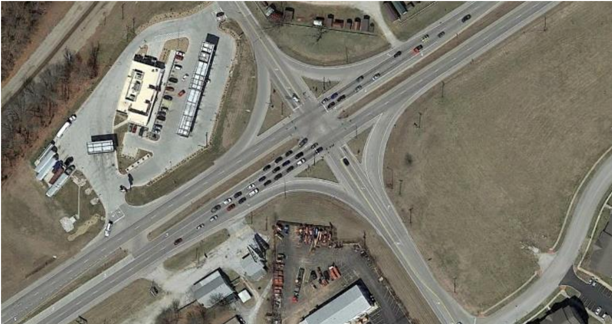
Existing intersection at US 60, Route MM, & Route M in Republic
