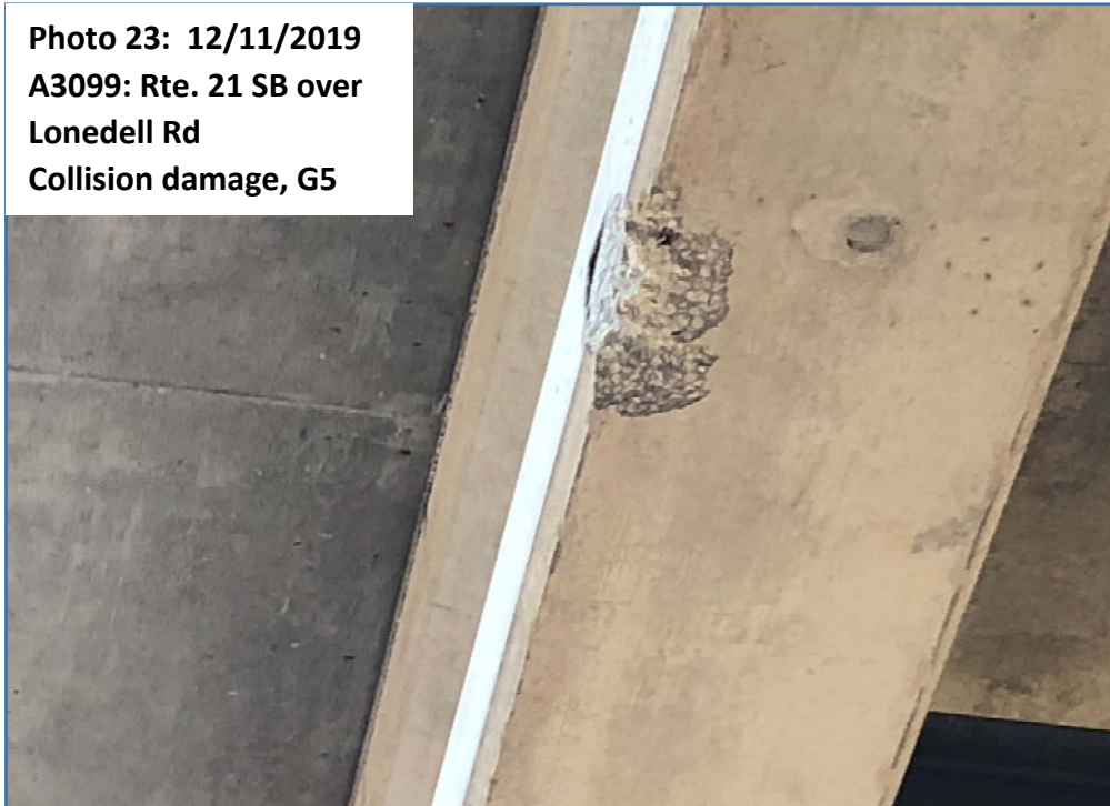
Photo 24: 12/11/2019 A3099: Rte. 21 SB over Lonedell Rd Collision damage, G5
