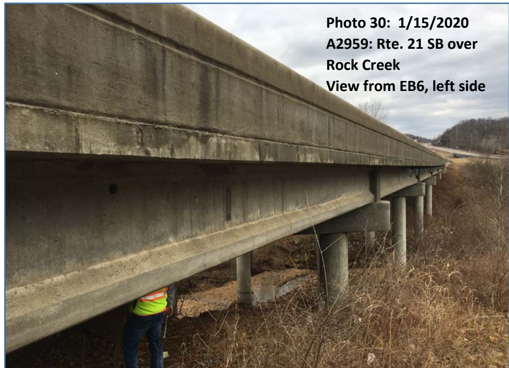
Photo 32: 1/15/2020 A2959: Rte. 21 SB over Rock Creek EB6, slope protection, under G1
