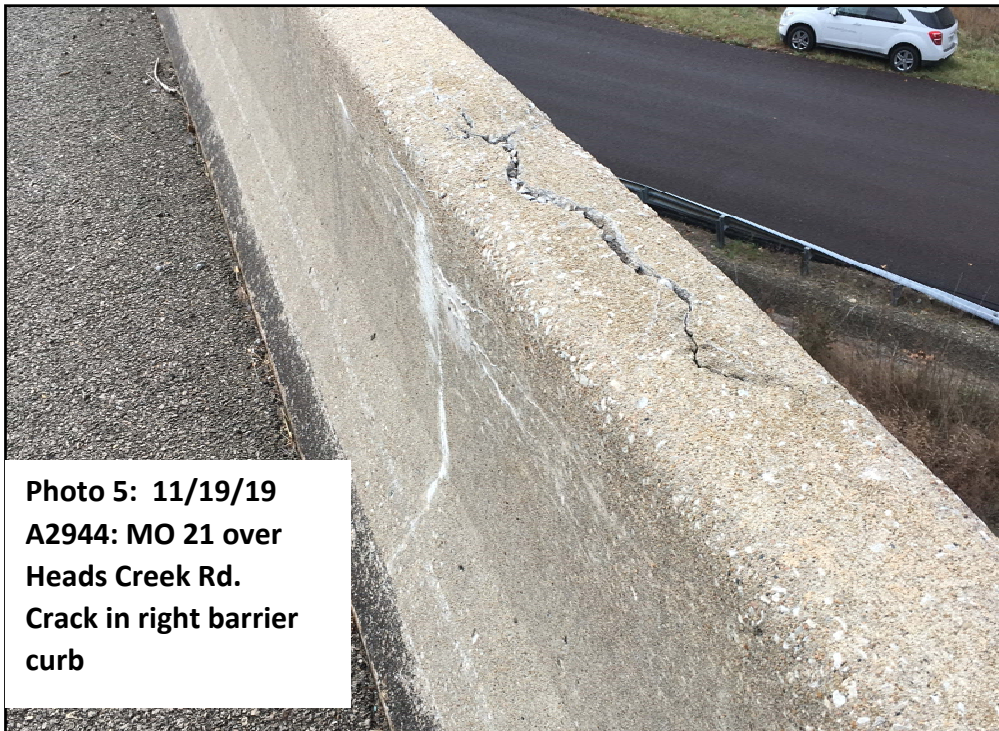
Photo 6: 11/19/19 A2944: MO 21 over Heads Creek Rd. 12' delam on west Crack in right barrier
